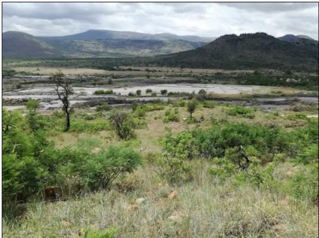
Photograph 5. Degraded paste tailings facility on the proposed WRD site
