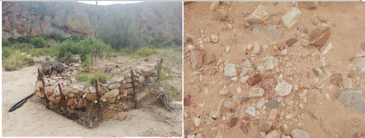
Bank stabilisation efforts
