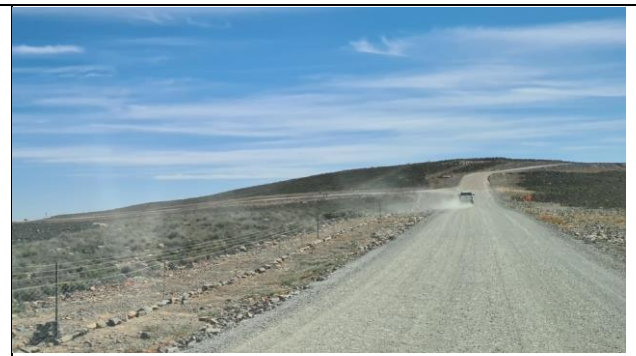
Figure 73: Typical WEF constructed access road.
