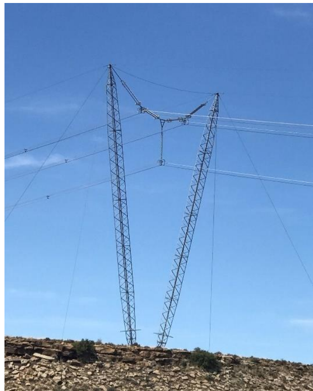
Figure 76: Pylon design that provide fewer opportunities for nesting sites.
