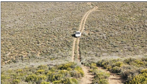
Figure 72: Typical two-track type farm road.
