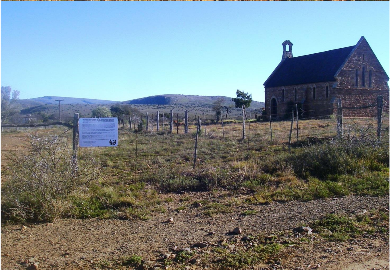
Plate C4 (3) – Site notice erected on the dirt road linking the R400 and Alicedale.
