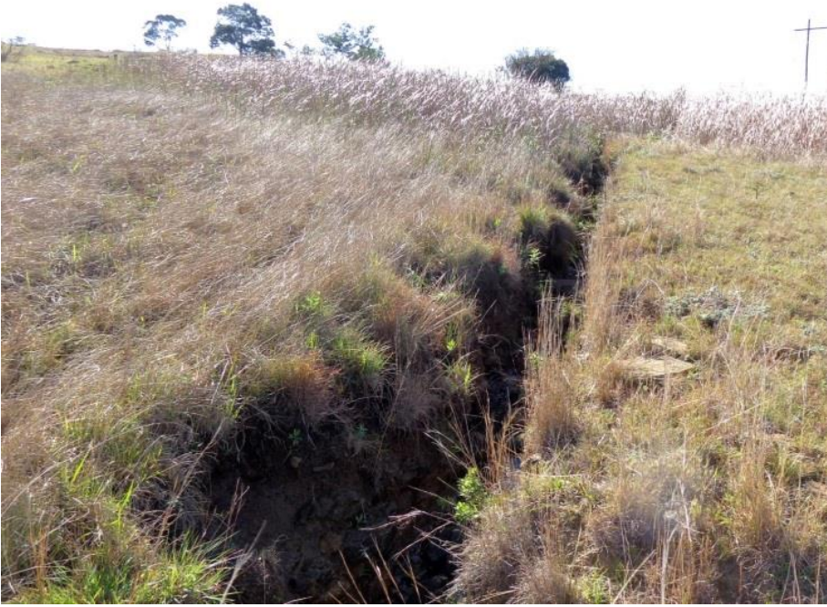
Figure 5.10: A section of the trench that was dug to direct water away from the discharge point
