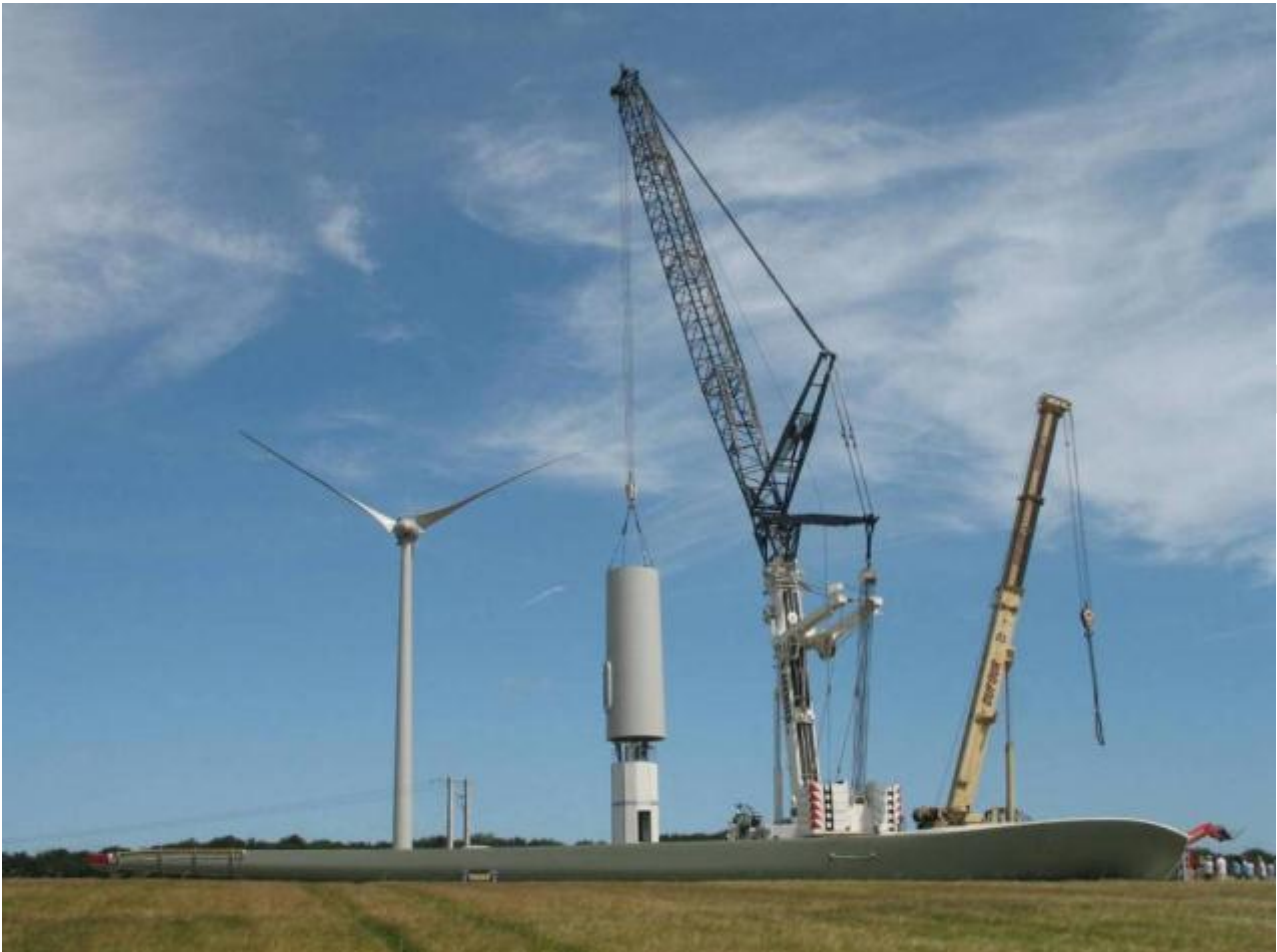
Plate 2-3: Assembly and erection of the tower sections using cranes
