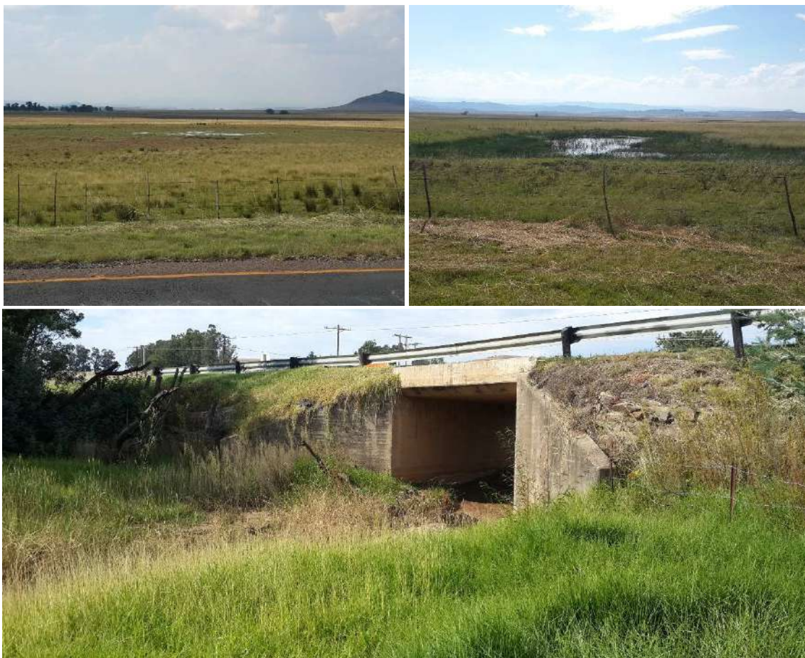
Photo Plate 3: Pan (top left), dam and moist grassland (top right), and major culvert over drainage line (bottom)
