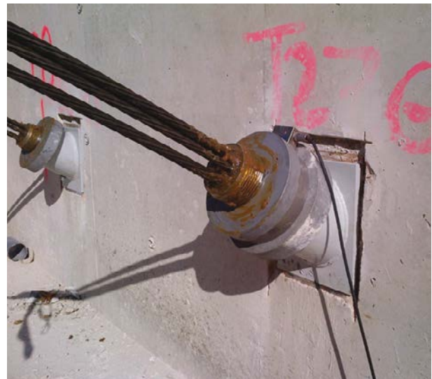
Picture 8.5: instrumented anchor head (© Freyssinet)
