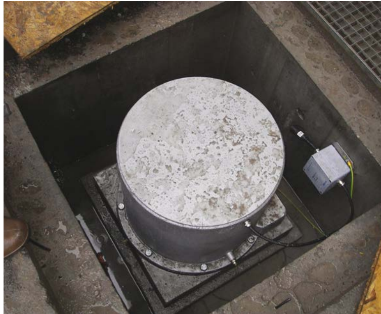
Picture 8.7: anchor head with a cap equipped with a control device (© François Morel-EDF)
