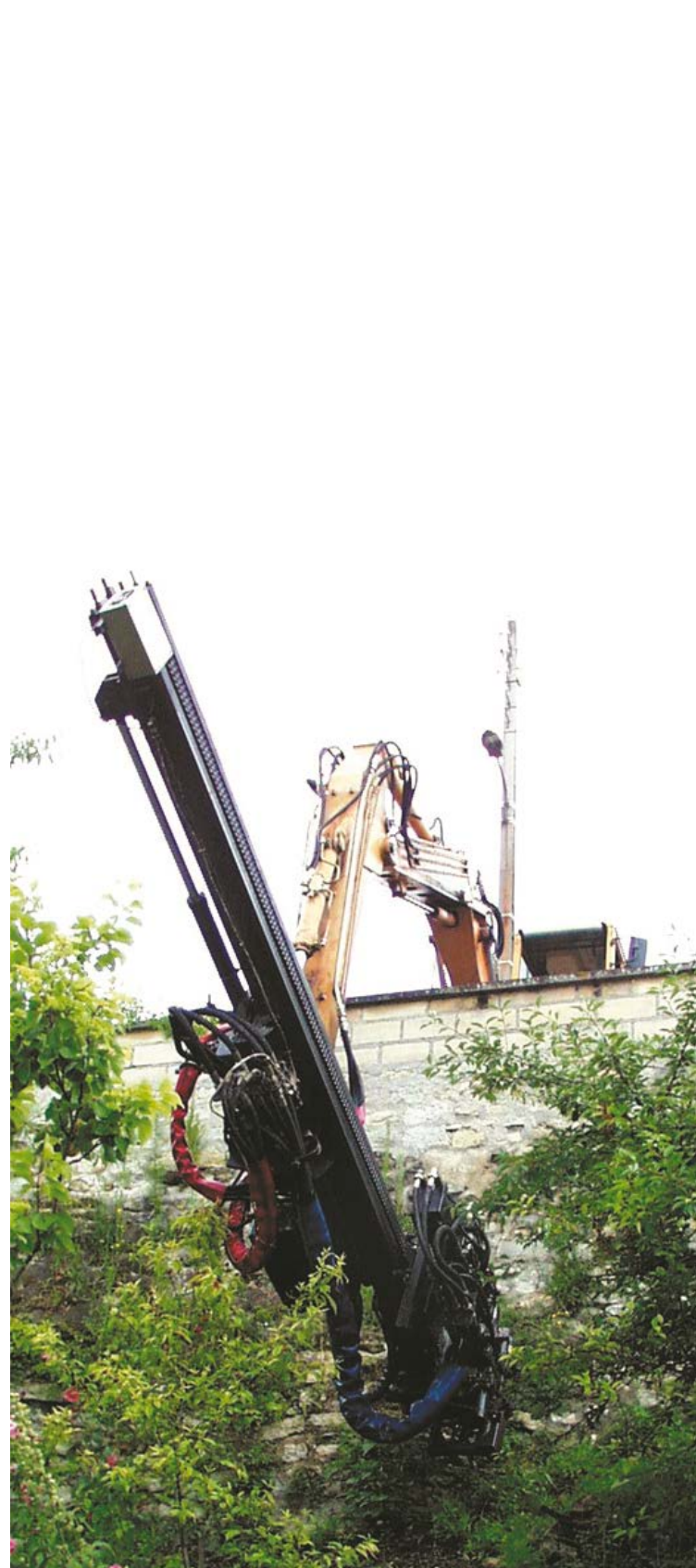
Picture 7.3: retromounted drilling rig (© Spie Fondations)
