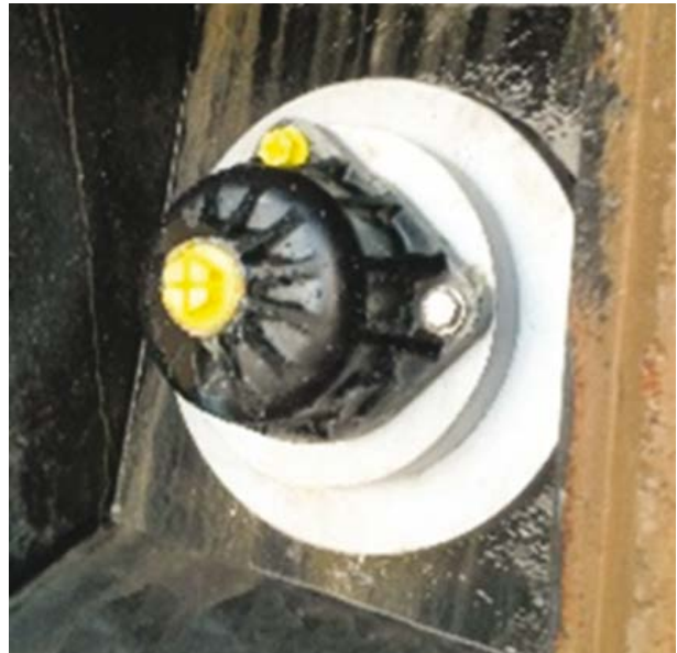
Picture 6.6: Anchor head with a type P protection (© Freyssinet)
