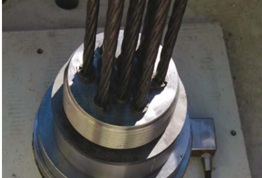
Picture 3.4a: Adjustable anchor head (© Freyssinet)
