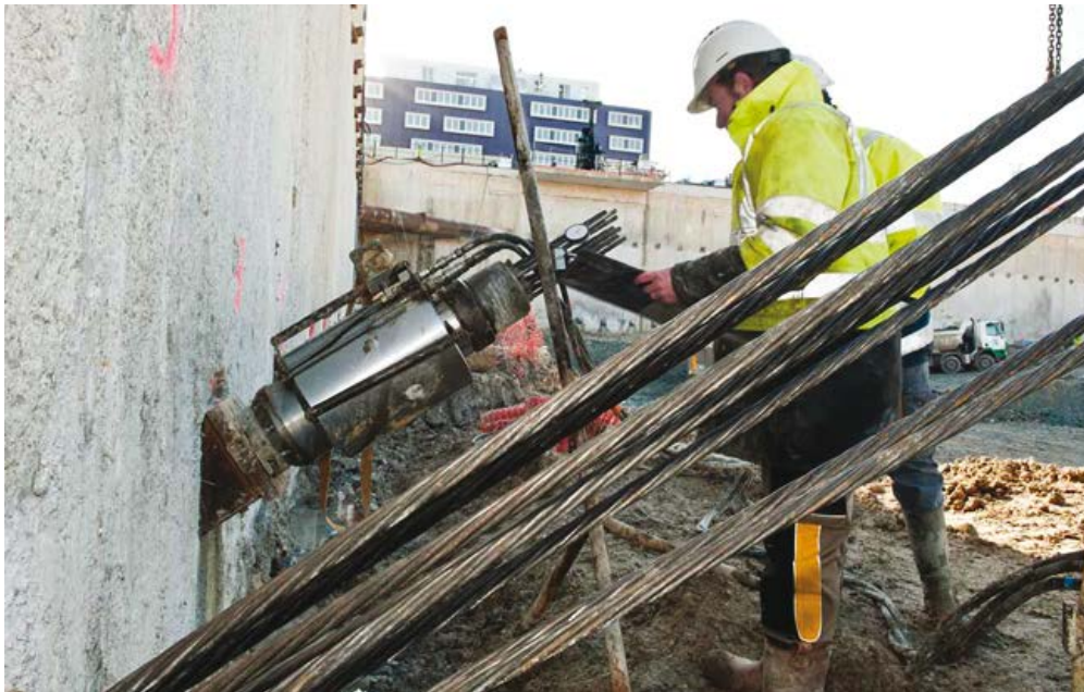
Picture 7.14: ground anchor stressing (© Sefi Intrafor)
