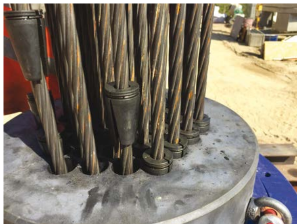
Picture 7.19a: Wedges being positioned (© Soletanche Bachy)
