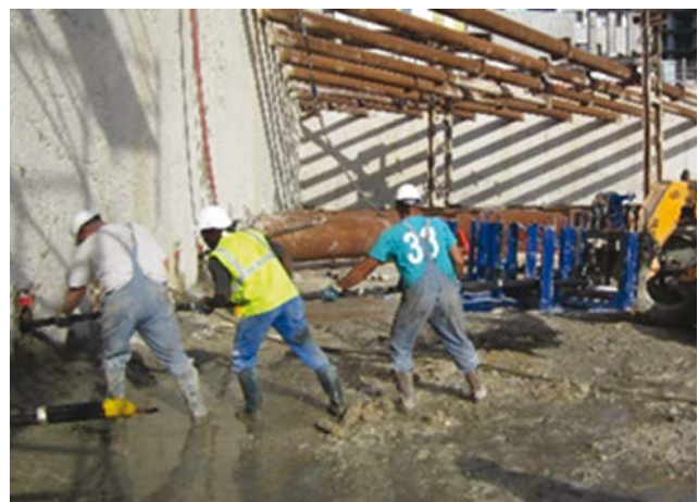
Picture 7.10b: ground anchor being unwinded into the borehole (© Freyssinet)
