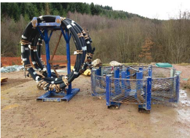
Picture 7.10a: (right) unwinder to facilitate the ground anchor installation and (left) conditioning gantry and winder (© Freyssinet)
