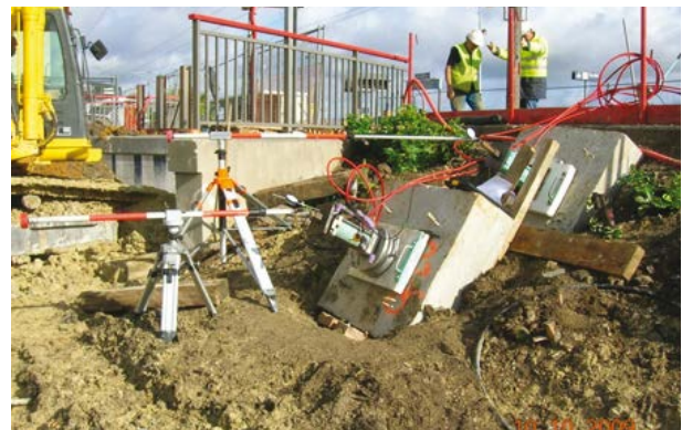
Picture 8.1a: concrete reaction block for a failure test (© SMG)
