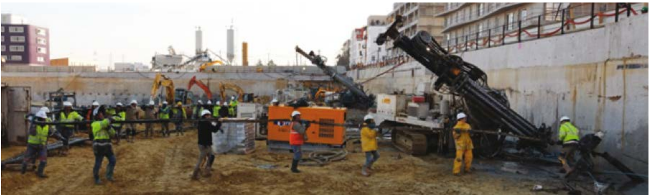
Picture 7.8: manual installation of a ground anchor (© Sefi Intrafor)
