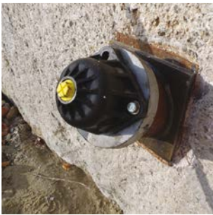
Picture 6.3: Anchor head with a type T protection (©Freyssinet)
