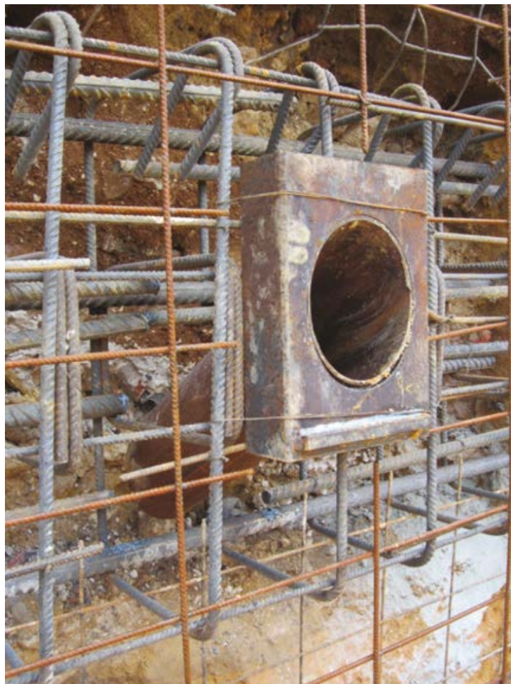
Picture I.2: Recess in a shotcrete wall (© Soletanche Bachy)
