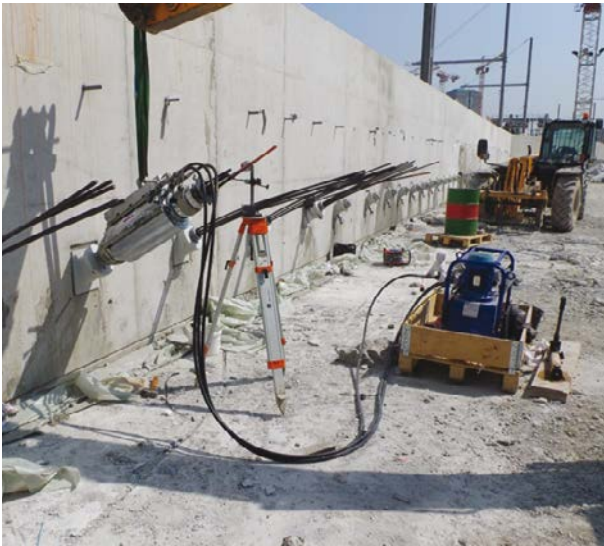
Picture 8.4: suitability test (© Soletanche Bachy)
