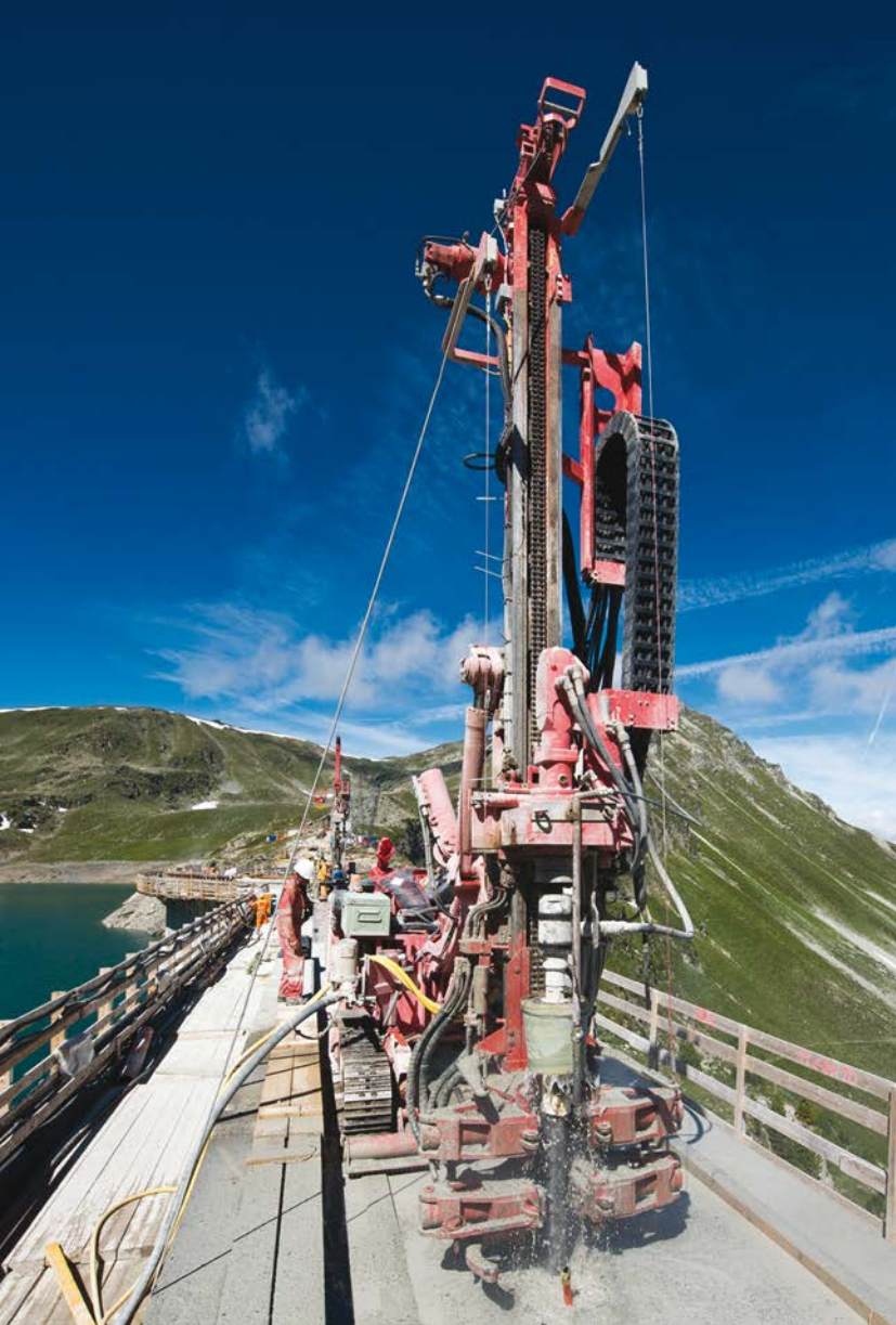
Picture 7.2: drilling rig on a dam (©Cédric Helsy- Soletanche Bachy)
