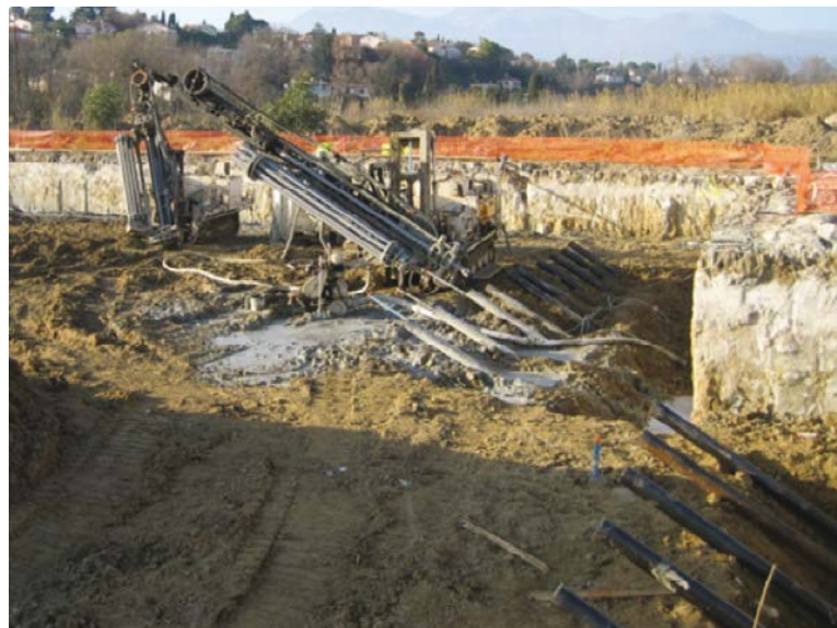
Picture 7.7: borehole with extension tubes (© Spie Fondations)
