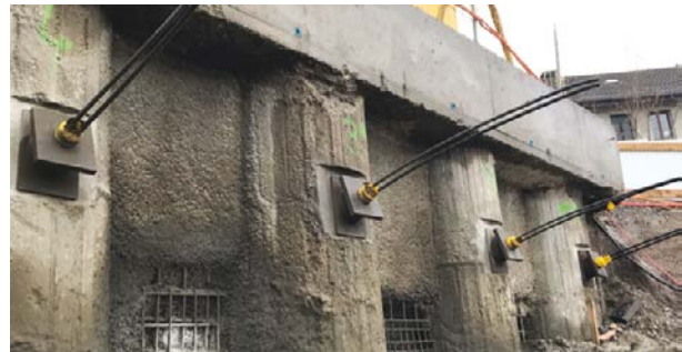
Picture 3.2: Support system reduced to a load-transfer block (on a Lutetian pile) (© Freyssinet)
