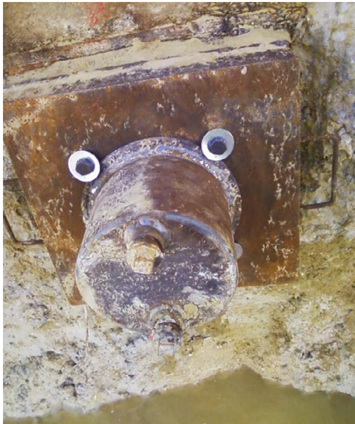
Picture 3.1: example of a protection cap (© Sefi Intrafor)
