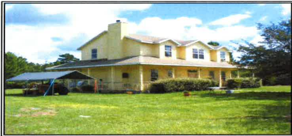
4. LOOKING NORTHEAST AT THE RESIDENCE
