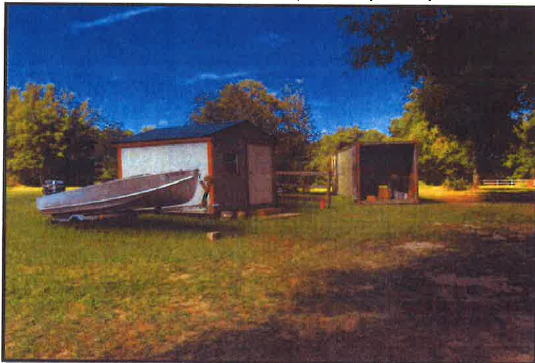
View of Shed B and Container B (see aerial p.14). (Photo #4)
