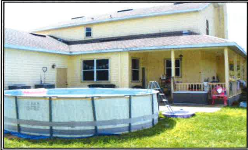
7. LOOKING SOUTH AT THE REAR OF THE RESIDENCE AND POOL
