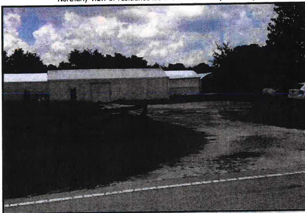
Northerly view of greenhouses from Ondich Road. (Photo #2)
