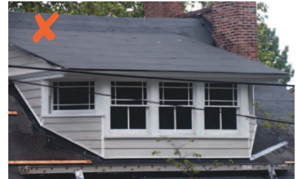
The HARB discourages the replacement of decorative shingles with other types of siding. The removal of the fish-scale shingles on this dormer has seriously compromised the historic integrity of the building.
