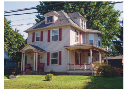
Charles W. Baum House (153 N. Main St.)
