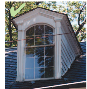
Storm windows, either glass or plastic, should fit the window opening. The arched shape of the dormer window on the left is hidden by the rectangular storm window.
