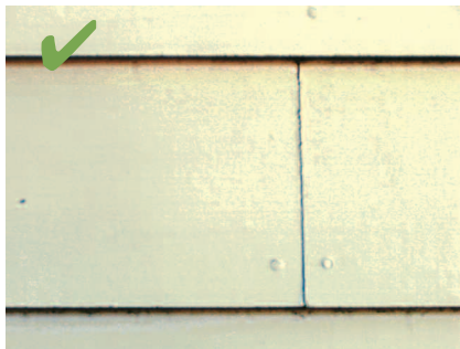
Rather than making siding appear more “authentic”, imitation wood grain (above) often makes the siding look very artificial. The HARB encourages the use of siding without imitation wood grain (below: cementitious siding).
