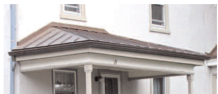
A metal porch roof.
