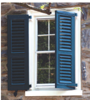
The photo at left shows the proper placement of shutter louvers; the louvers should shed rain when they are closed. Louvered shutters were originally designed to protect against the weather while permitting ventilation.
