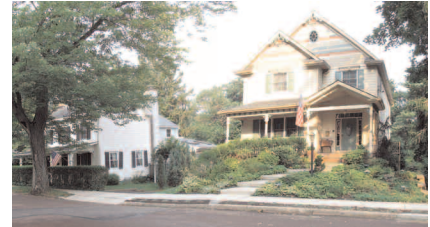
The infill house on the right has an artificially raised first floor. The HARB recommends that infill buildings have the same entrance level as their immediate neighbors. This does not mean that all buildings on a block must have raised porches or no porches at all, just that the natural grade level should not be raised excessively.
