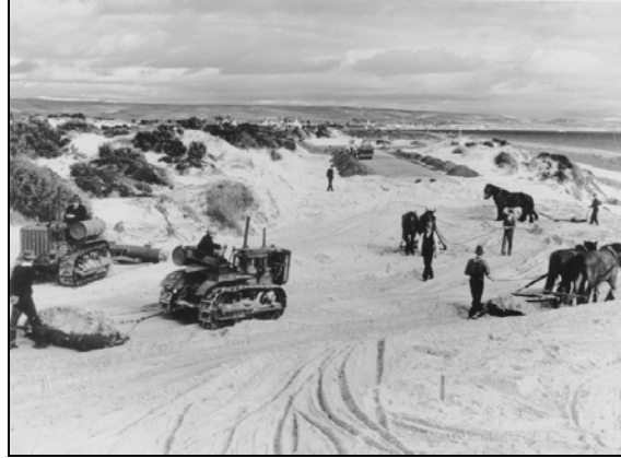
Figure 4: 1937 - Torrens Outlet Construction, Looking South
