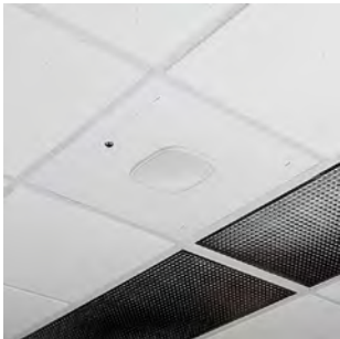
Enclosure with Cisco 9130 Door
