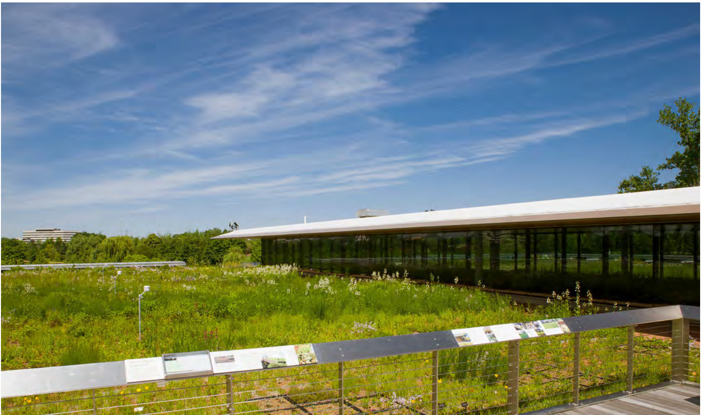
South green roof
