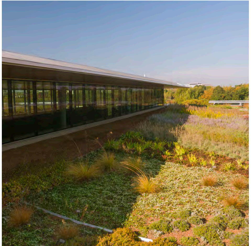
Shadow line on north green roof in late summer-early fall
