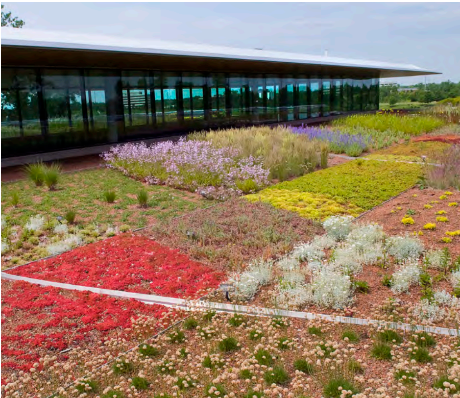
Sedum strip on north green roof
