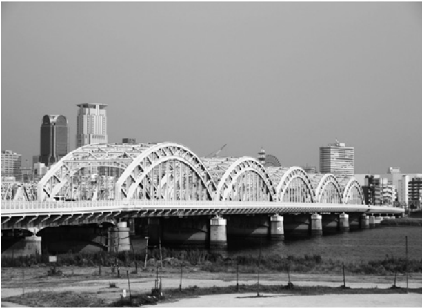
Fig. 1 Juso Bridge (Osaka)
