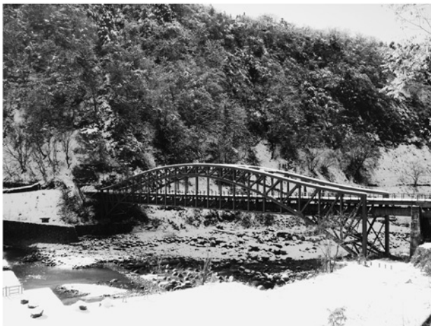
Fig. 5 JogANJI Aqueduct Bridge (Toyama)
