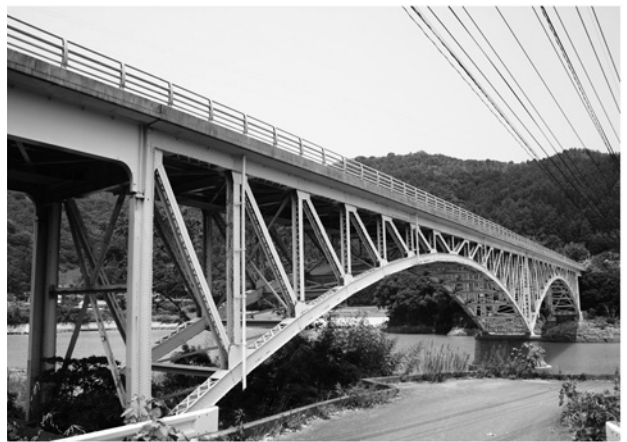
Fig. 4 Mimitsu Bridge (Miyazaki)
