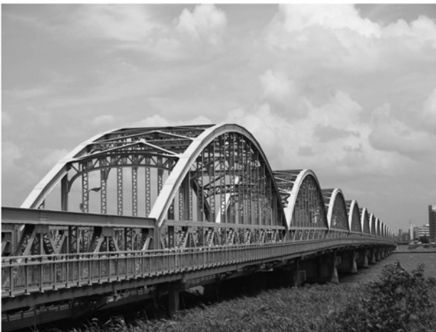
Fig. 2 Owari-Ohashi Bridge (Aichi)
