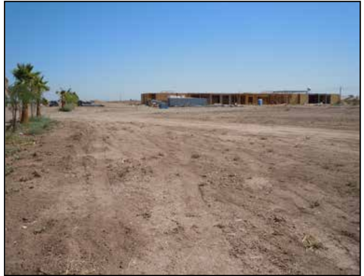
Photo 8. Southern Portion of Parcel: Graded barren areas with the partially-built building within the PSA. Photograph taken facing north.
