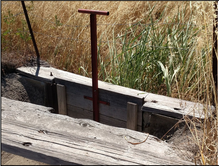
Photo point 9a: Irrigation gate looking south from cement ditch to vegetated ditch on property. Photo taken June 20, 2019.
