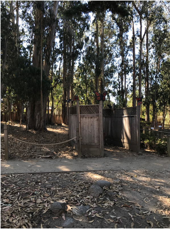
A. PERMANENT RESTROOM LOCATION (AS SEEN FROM PATH FACING SOUTHWARD)
