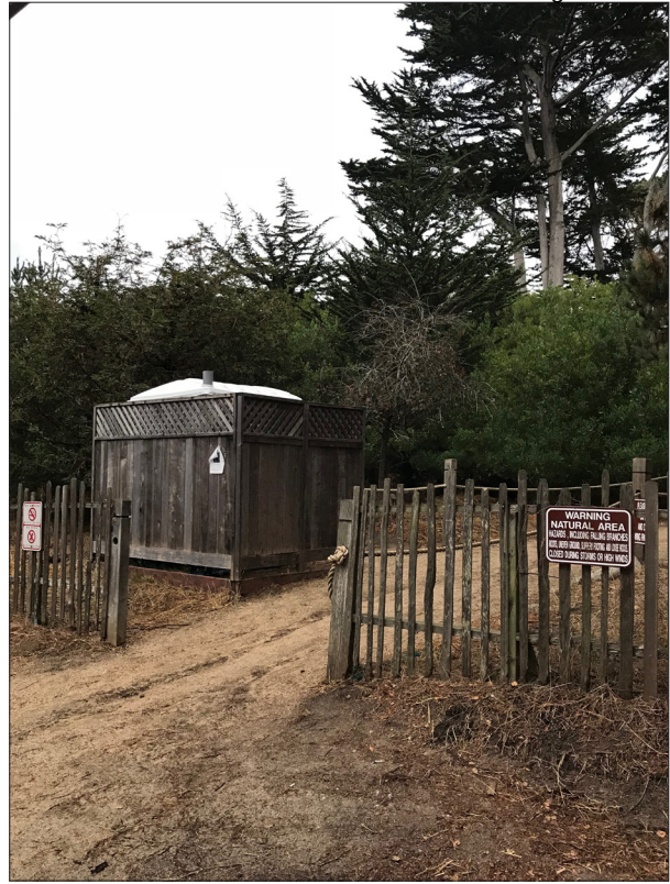
B. PORTABLE RESTROOM LOCATION (AS SEEN FROM GROVE ACRE AVENUE FACING EASTWARD)
