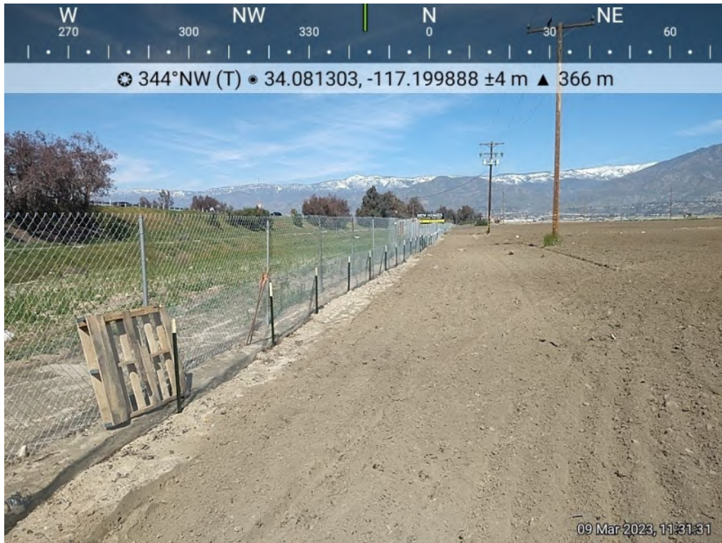
Photograph 3: View of utility poles and chain-link fence on the site adjacent to Highway 210.
