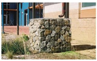
Gabbion for Energy Dispersion (i.e., erosion control)
