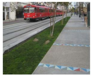
Figure 11: Vegetated Filter Strip (Source: 3 **Rivers Wet Weather)**
