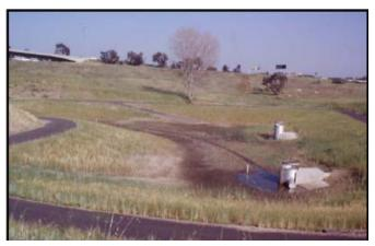
Figure 1: Infiltration Basin (Source: CASQA Stormwater BMP Handbook)
