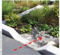
Figure 4-2: This standard curb cut at parking lot rain garden has 45 degree chamfered sides.
