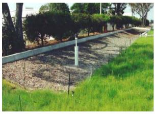
Figure 2: Infiltration Trench (Source: LA LID Manual)
