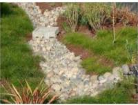
Figure 4-1: Cobbles in this stormwater treatment measure in San José help prevent erosion.
