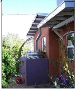
Figure 8: A rainwater capture and reuse system on a residential home. (Photo: Kennedy/Jenks Consultants)
