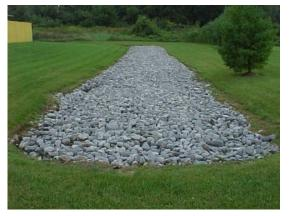
Infiltration Trench Source: Contech Engineered Solutions
