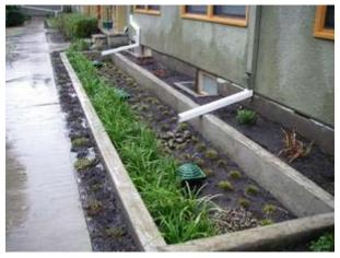
Figure 7: Stormwater Planter (Source: Portland BES)
