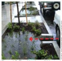
Figure 4-5: The side wings of this standard curb cut help retain the side slope grade on each side of the curb cut opening.
