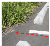
Figure 4-8: Stormwater runoff enters the stormwater facility through the 3-foot space between these wheelstops. The design could be improved by providing more of a drop in grade between the asphalt and landscape area.
