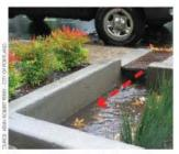
Figure 4-11: A grated curb cut allows stormwater to pass under a pedestrian walkway to the stormwater facility.
