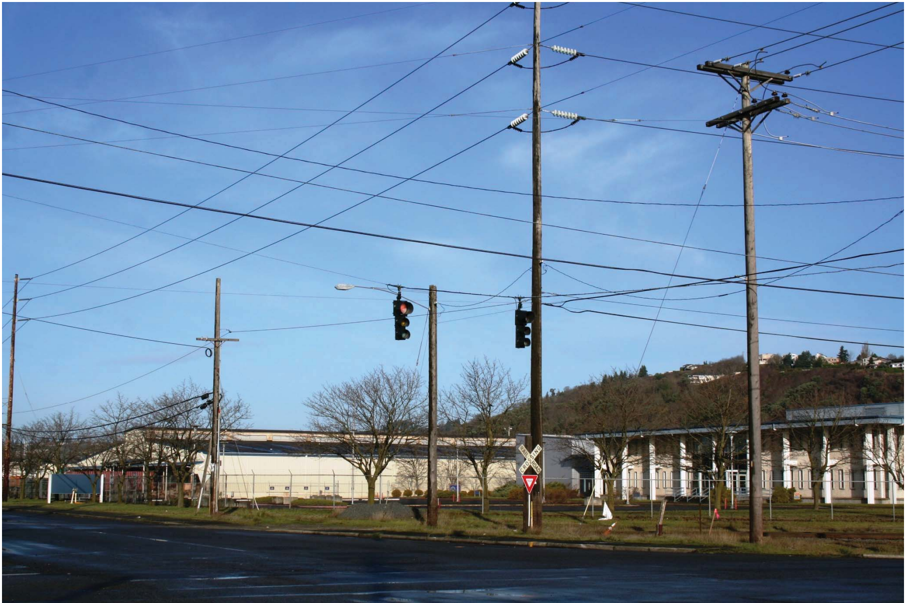
KOP 4a: View to the northwest of the Tacoma LNG Facility site from the corner of East Alexander Avenue and East 11th Street.
