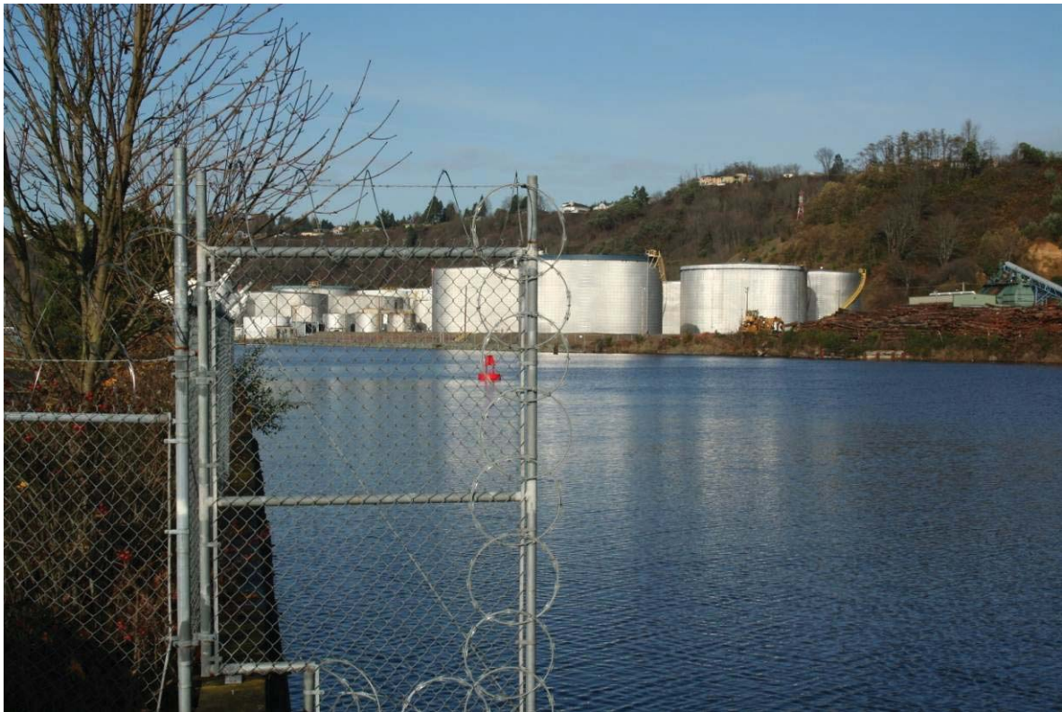
Location 6. Along edge of Hylebos Waterway looking west toward tank farm.
