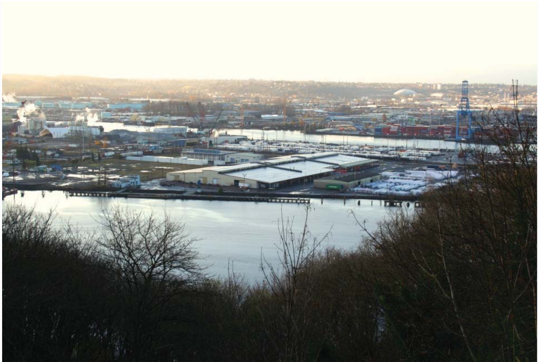
KOP 1a: Existing view to the south of the Tacoma LNG Facility site from the sidewalk of Browns Point Boulevard north of McMurray Ravine.
