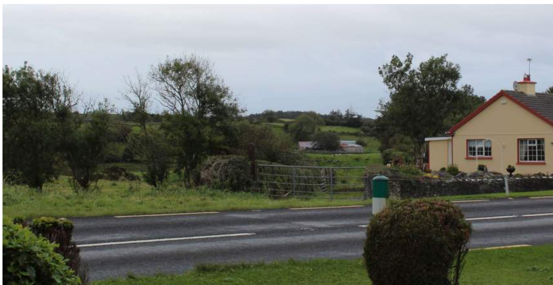
Plate 5-13 Route of former railway corridor in front of dwelling (adjacent to the N67 east of Ennistymon)
