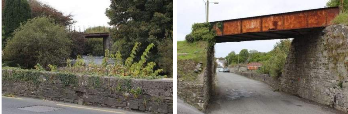
Plate 5-18 & 5-19 Remnants of railway bridges in Ennistymon, background of Plate 5-17.
