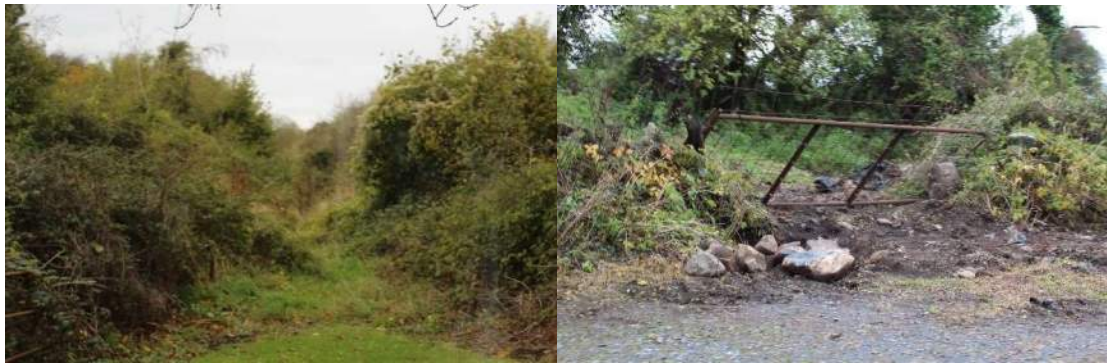
Plate 5-6 & 5-7 Route of the disused railway line with trees and groundcover vegetation visible from the local roads at Drumcavan, and at Kilkee East southeast of Corofin
