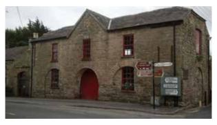
Mountshannon Market house was built around the year 1740. Built with exposed rubble walls, it is a detached three-bay two-storey building with gabled central bay and slated half-hipped roof. There are three arched openings on the ground floor, forming an arcade, two of which were blocked up around 1920.
