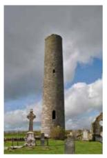
The round tower of Inis Cealtra is without a roof and it is possible that it was never completed. Excavations and restoration work carried out in the 1970s, failed to uncover any stones that may have belonged to a round tower's cone-cap. Although they may have been reused in other buildings, the legend that the tower was left "unfinished" because the
