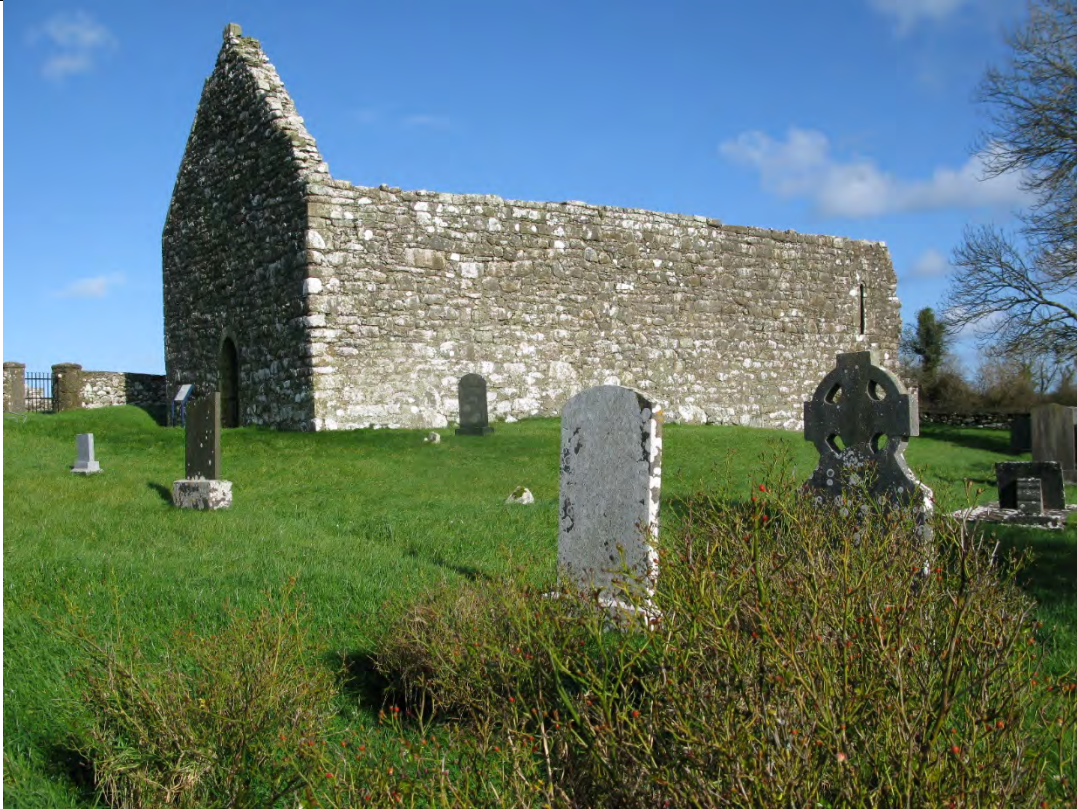
Image showing south elevation to St Mary's Church.
