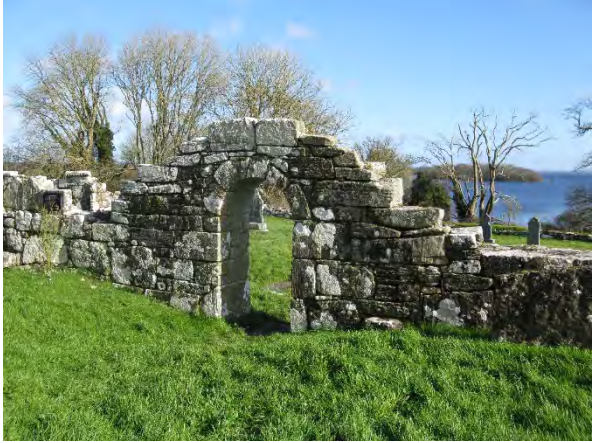
External view to entrance arch to Saints' graveyard within main churchyard.
