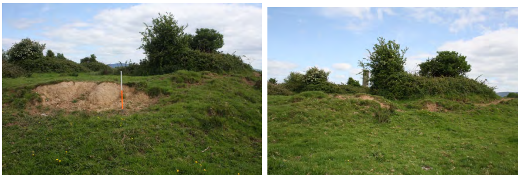
Figs 69 and 70: Damage to outer enclosure of St Michael’s caused by cattle (Photos: B. McCarthy)
