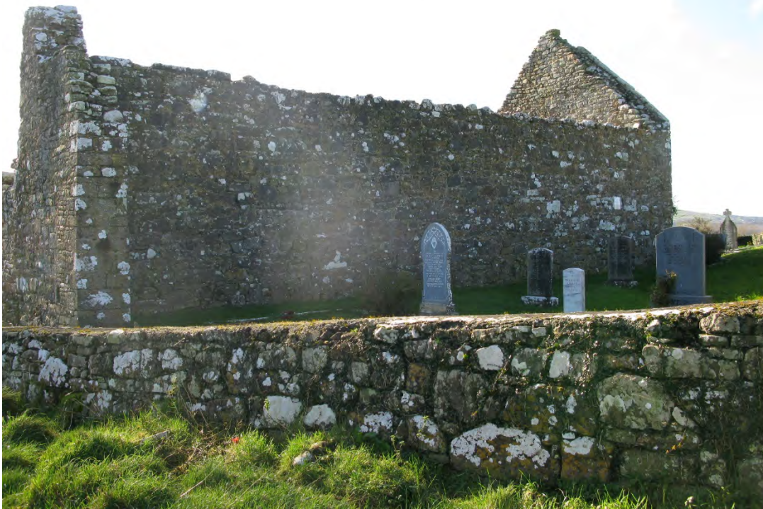
Image showing south elevation to St Mary's Church.
