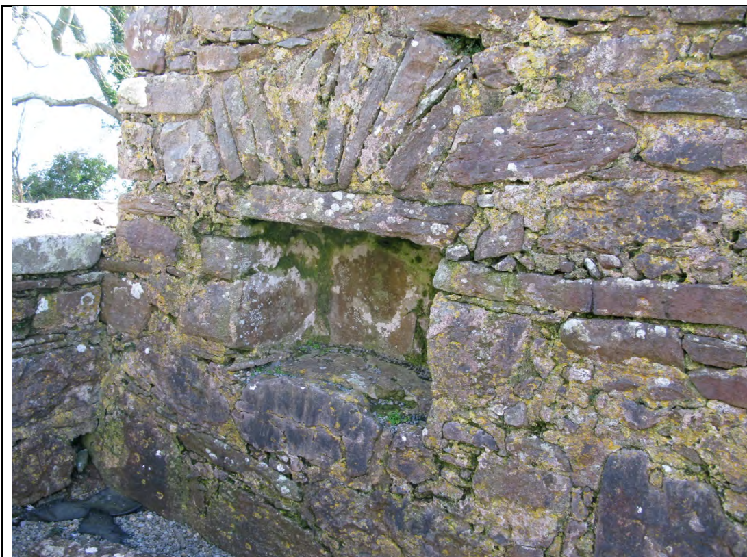
Detail showing ambry to south east wall.
