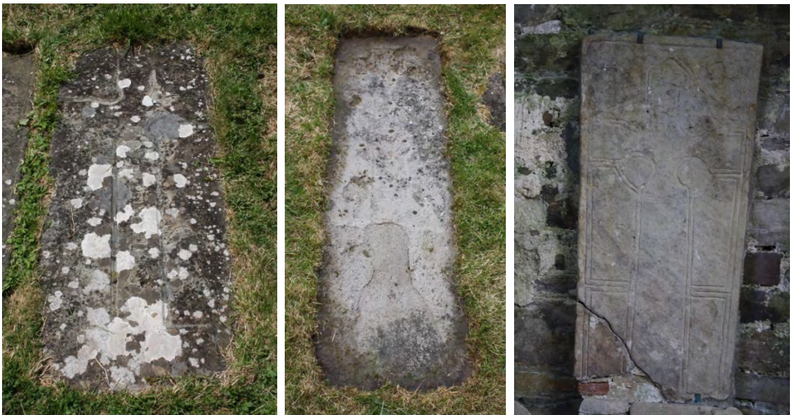
Figs 74-6: Cross-inscribed grave-slabs suffering from delamination: left and centre in the Saints' Graveyard, with RMPs CL029-009096- and CL029-009101-; right in St Caimín's Church with RMP CL029-009106- (Photos: C. O'Leary)
