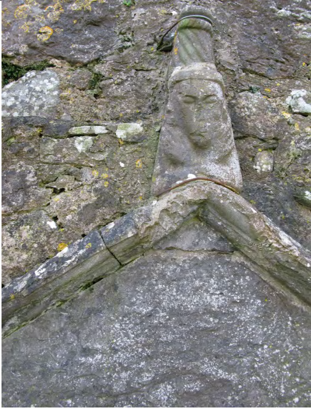
Detail showing apex of plaque. Note rusting wire used to secure item.
