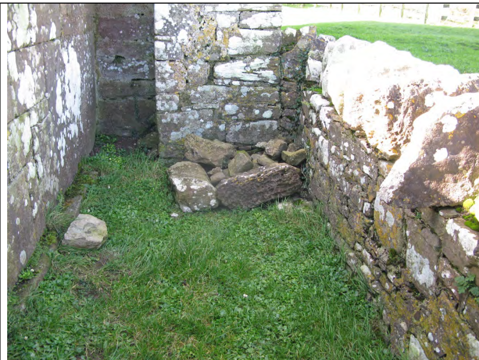
Loose stone to base of wall between north chancel and enclosing wall.
