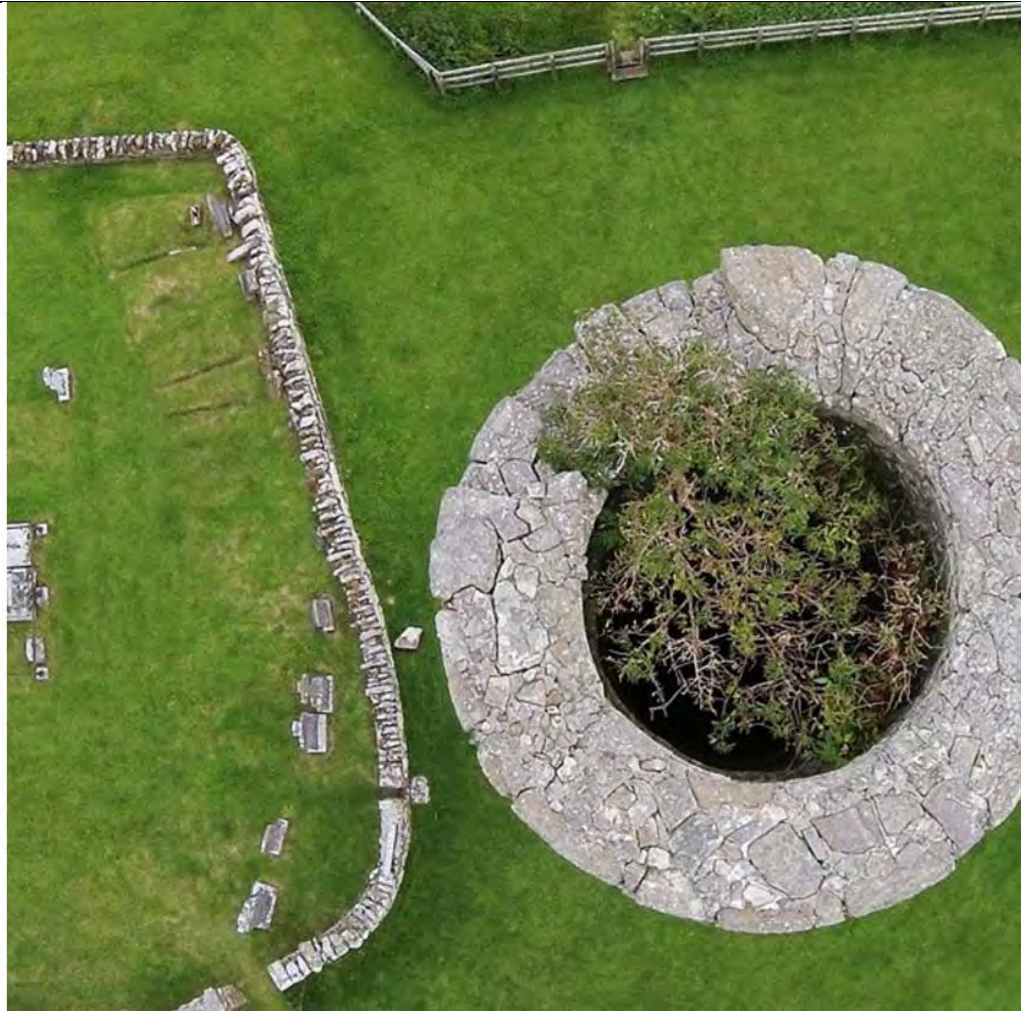
Image showing tree growth in tower and dislodged stone. (Image taken by Eoin O'Hagan)
