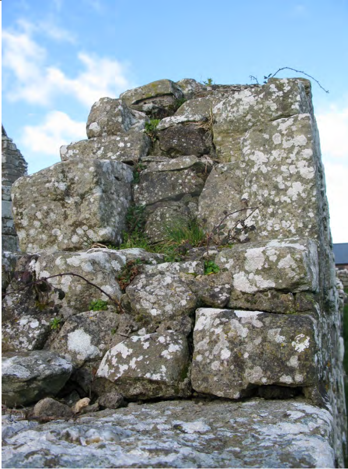
Image showing open joints with vegetative growth including the deeply rooting Rubus fruticosus (blackberry).
