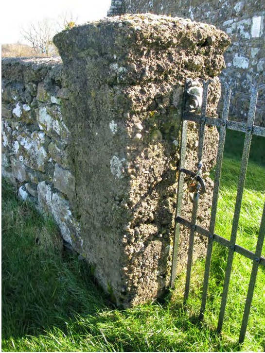
Image showing poured concrete piers to graveyard entrance.
