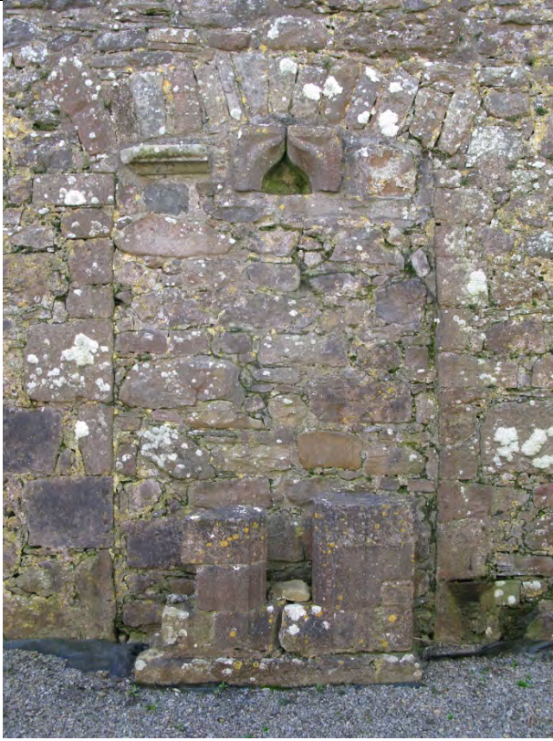
Image showing blocked up door opening to south wall with various carved stone pieces.
