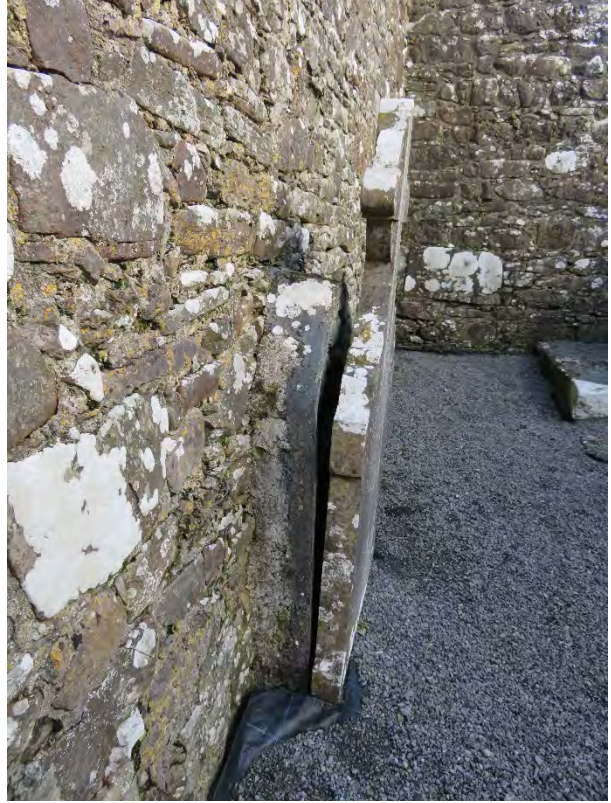
Cross mounted headstone leaning out of position on north wall of St Mary's Church.
