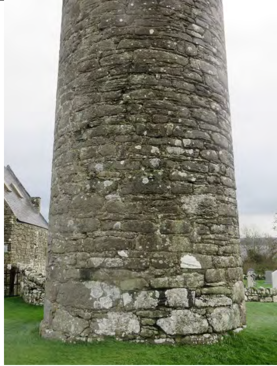
Image showing base to west elevation.
