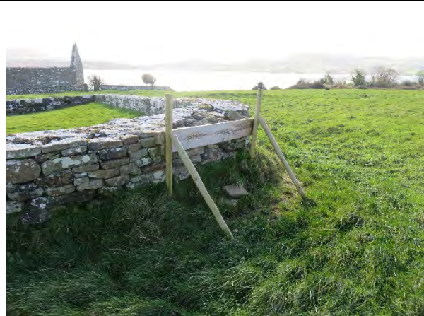
Image showing protection to North West corner of St Brigid's enclosure.
