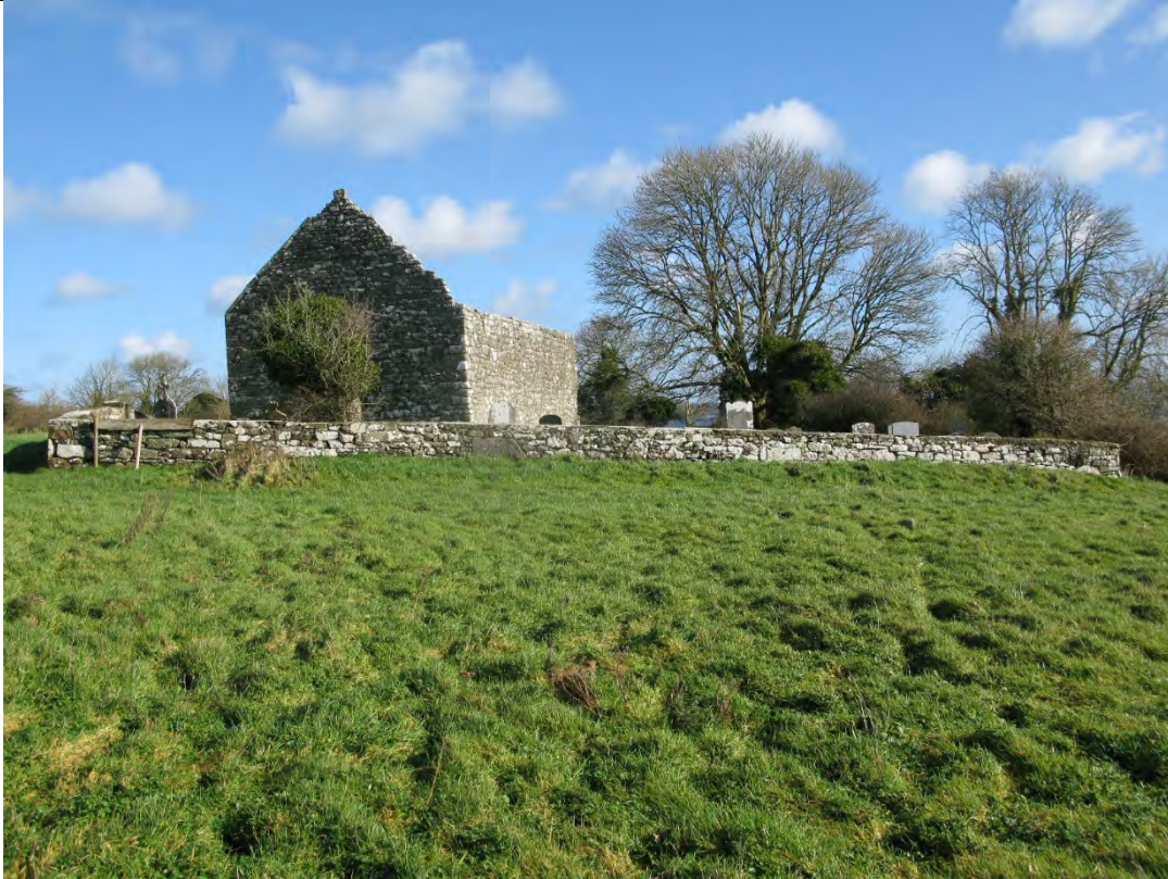
Image showing west elevation to enclosing wall to St Mary's Church and graveyard.
