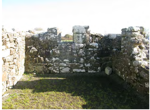
Interior east wall to St Brigid's Church.
