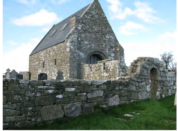
View showing internal elevation to west wall Saints' graveyard.
