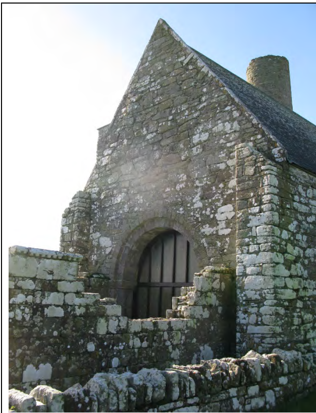
Image showing north elevation to chancel.
