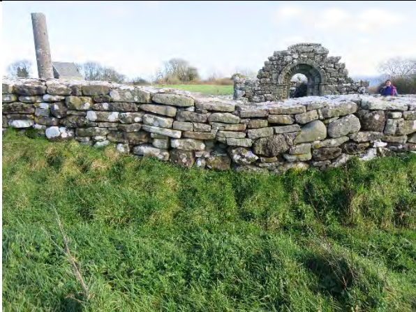
Image showing external west enclosure.
