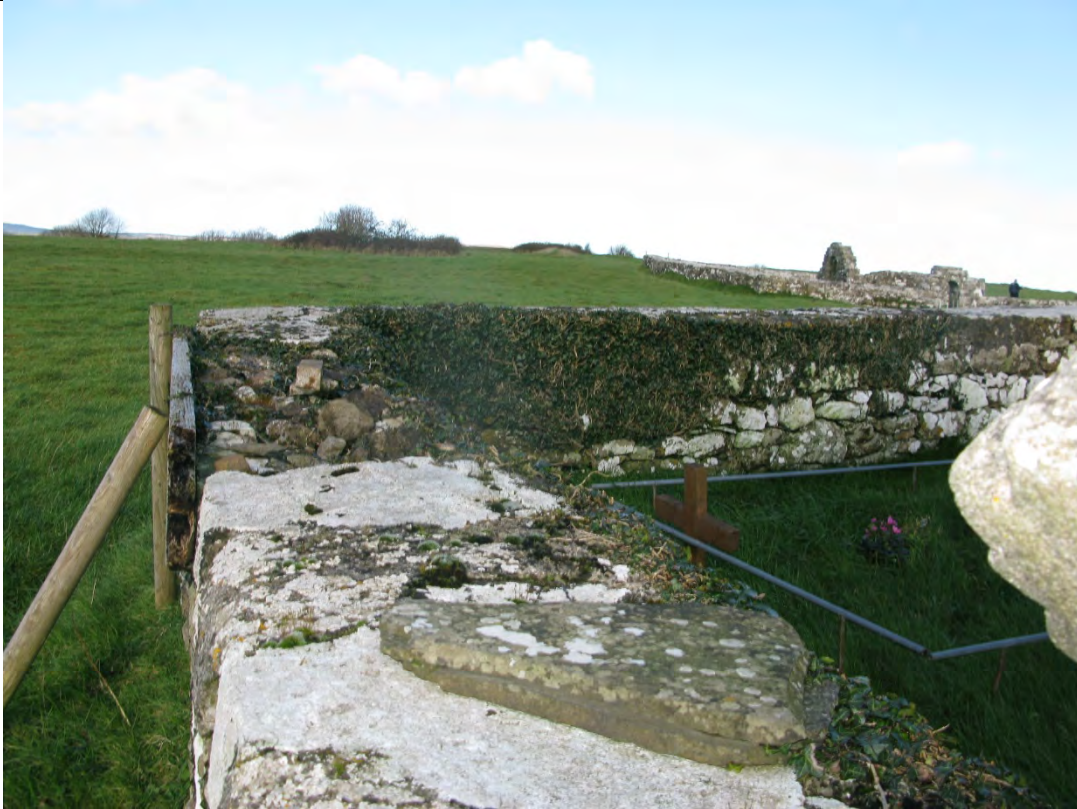
Detail showing shoring and loss of stone to the north west corner of the enclosure wall.
