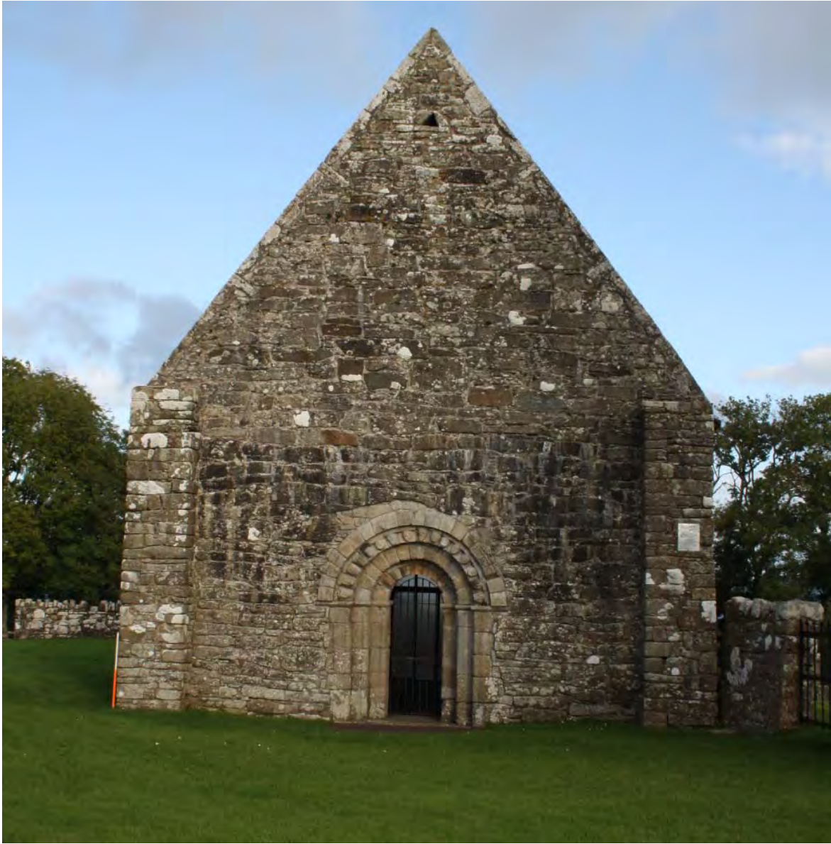
Fig. 1: W gable of St Caimín's Church (Photo: C. O'Leary)
