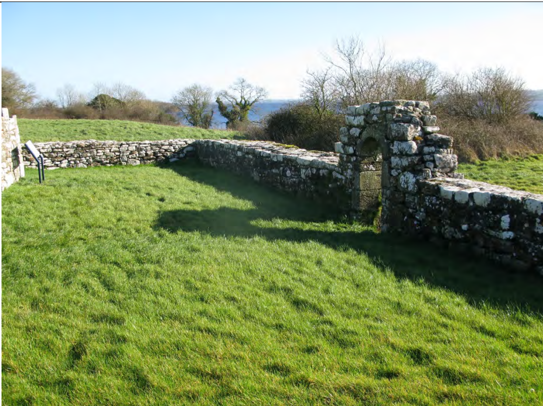
Internal south wall to St Brigid's enclosure.
