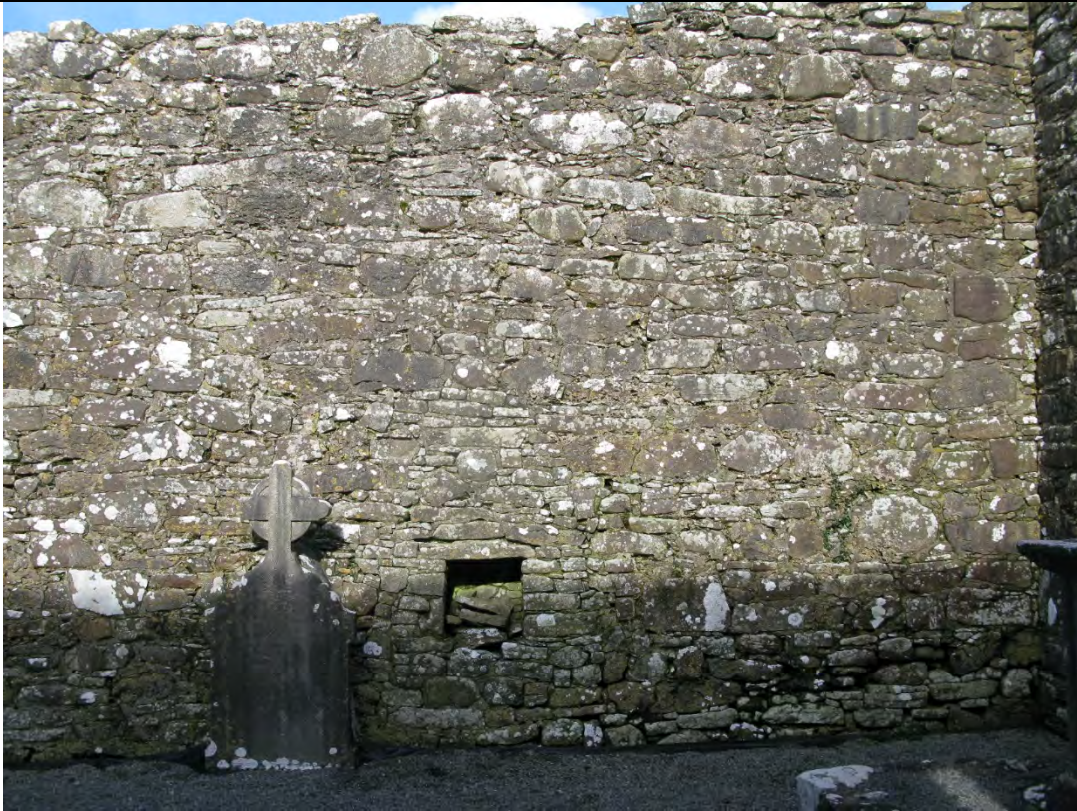
Internal north wall of St Mary's Church.
