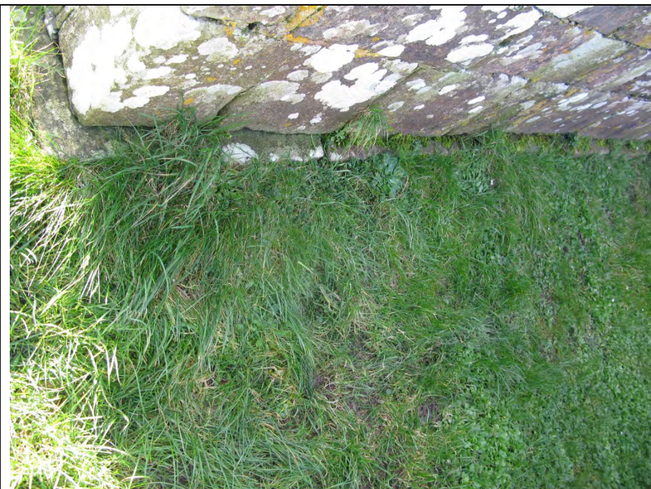
Loose stone to base of wall between north chancel and enclosing wall.
