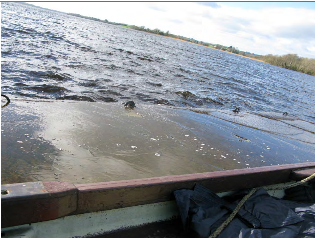
Surface to outer section of pier. Note horse shoes for mooring boats.
