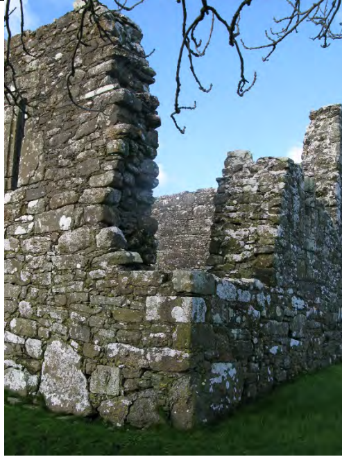
Detail showing south east corner of church.
