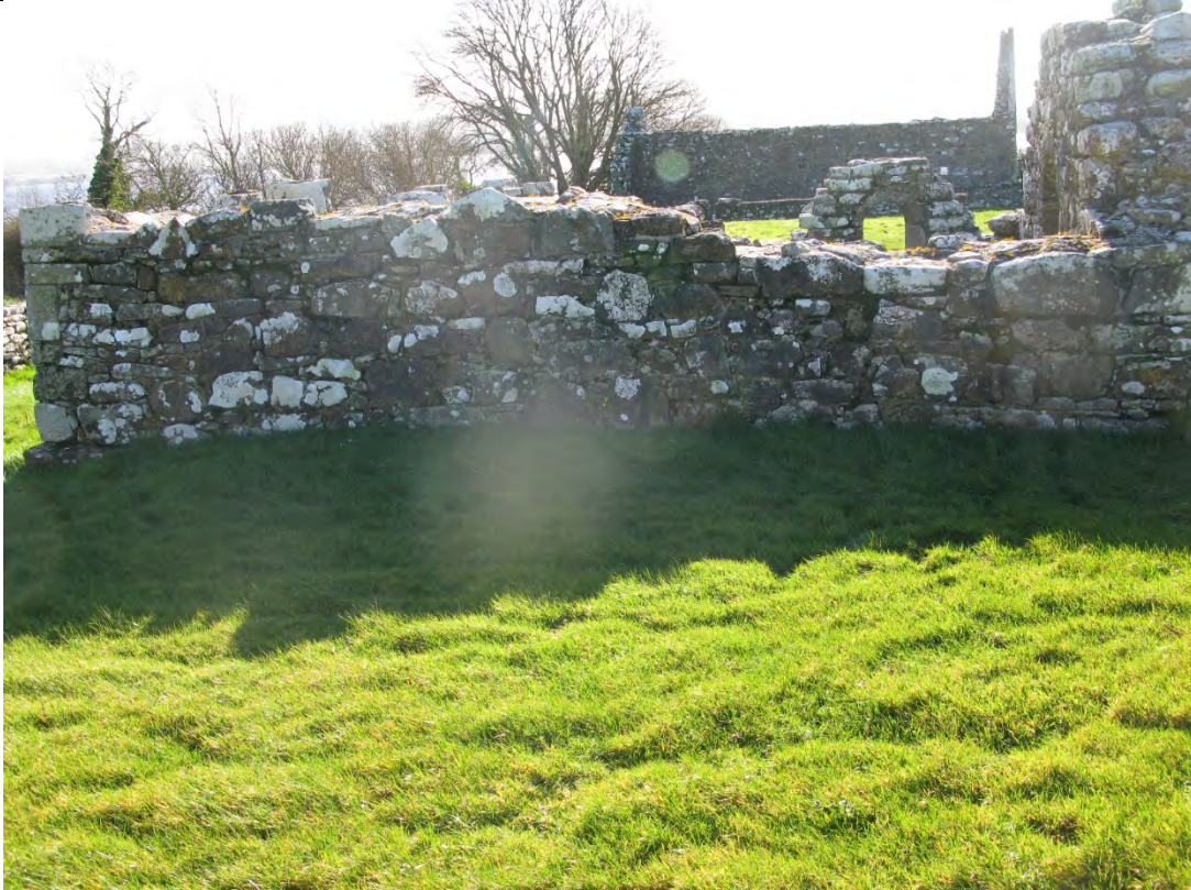
Image showing external north wall to St Brigid's Church.
