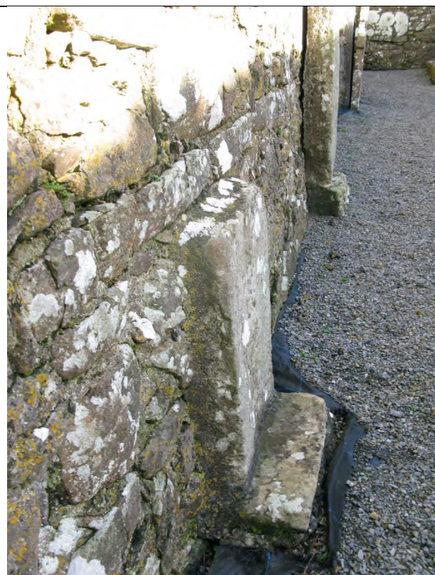
Detail showing cement bound grave slabs.
