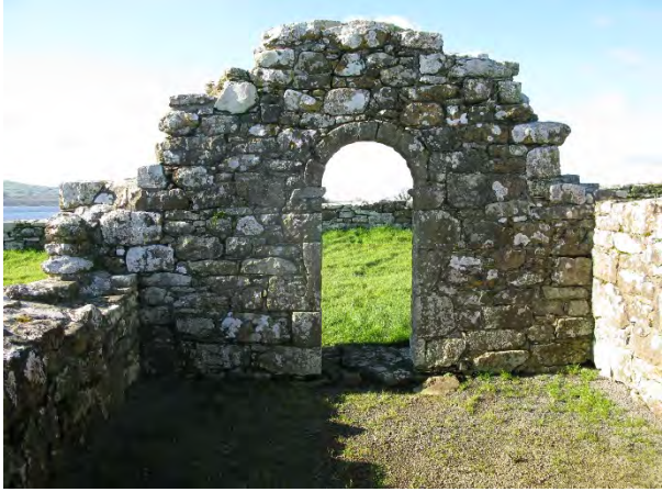
Interior west wall to St Brigid's Church.
