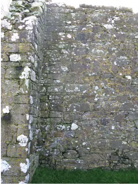
4.8.1.1.1 Image showing buttress to north east corner.
