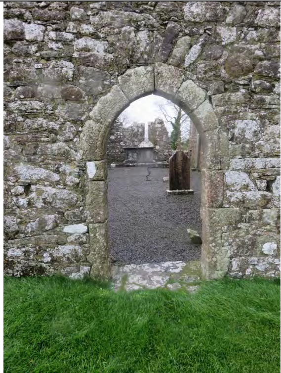
Detail showing door surround to entrance to St Mary's Church.
