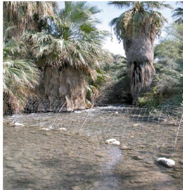
Figure B.5.1. Downstream view of channel within segment 5. Channel has been widened and coarse material placed for a vehicle and water pipeline crossing at this location. Channel is much narrower and contains fine grained material both above and below photo location.
