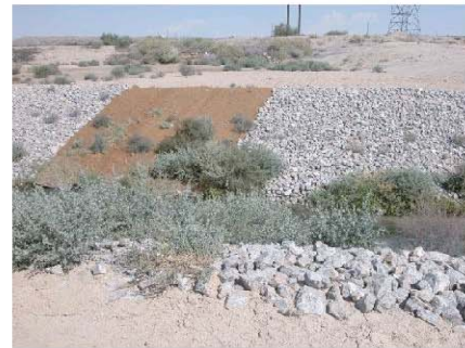
Figure B.1.6. Kern River pipeline crossing downstream from Reid Gardner Station.
