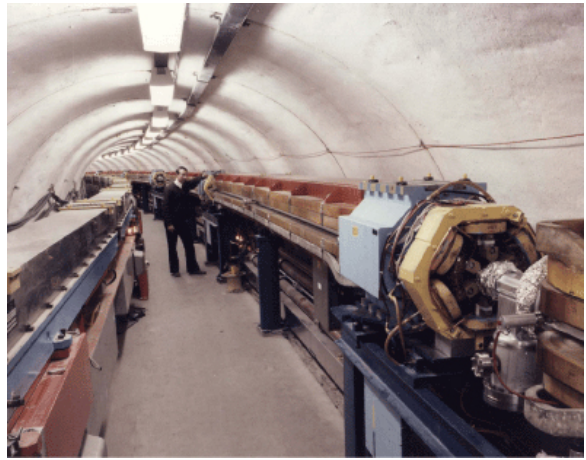
(b) Inner view of the tunnel.
