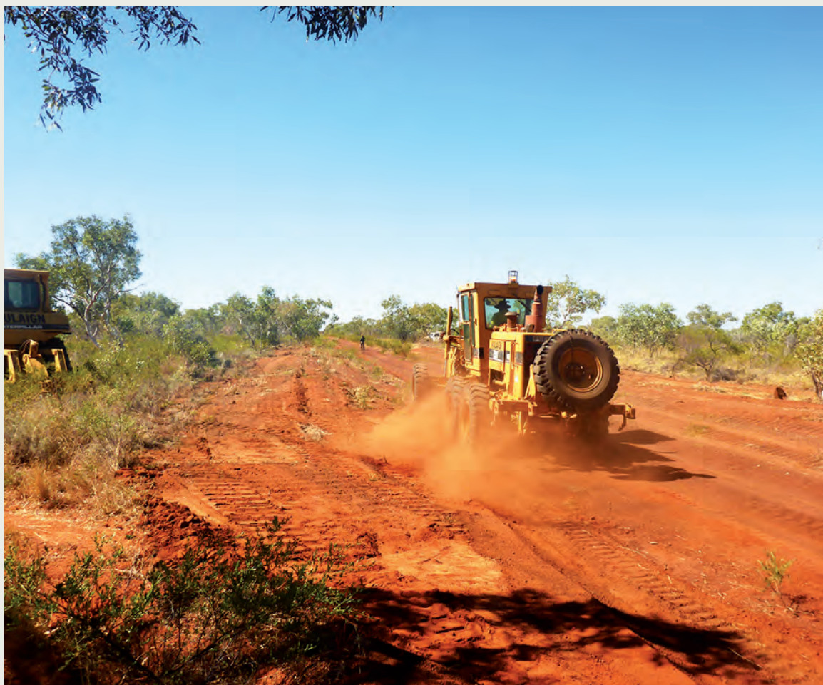
Wulain grader repairing erosion damage on Duck Ponds track in 2015
