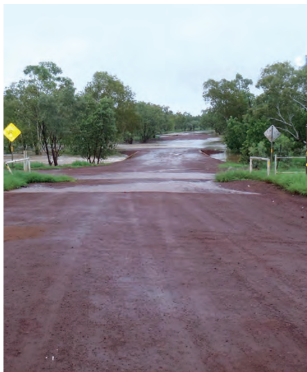
Flood waters over Lajamanu Road
