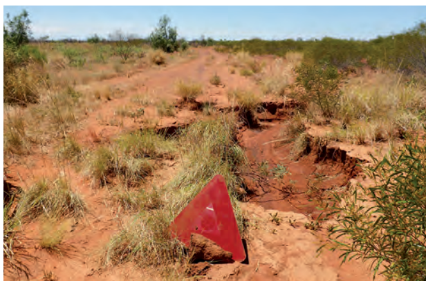
Erosion damage on track through Duck Ponds area
