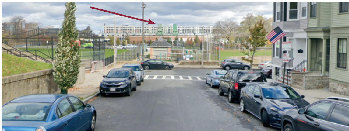
The Massachusetts Bay Transit Authority's M Street Jets peaker plants sit near ball fields, a park, and a dense urban neighborhood. The red arrow points to the jets' emissions stacks. PHOTO: GOOGLE EARTH
