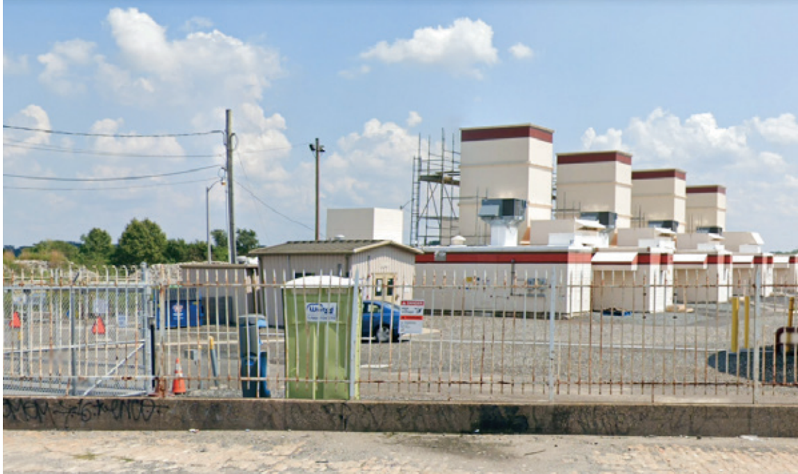
Street-level view of Delaware CT peaker plant in Philadelphia
