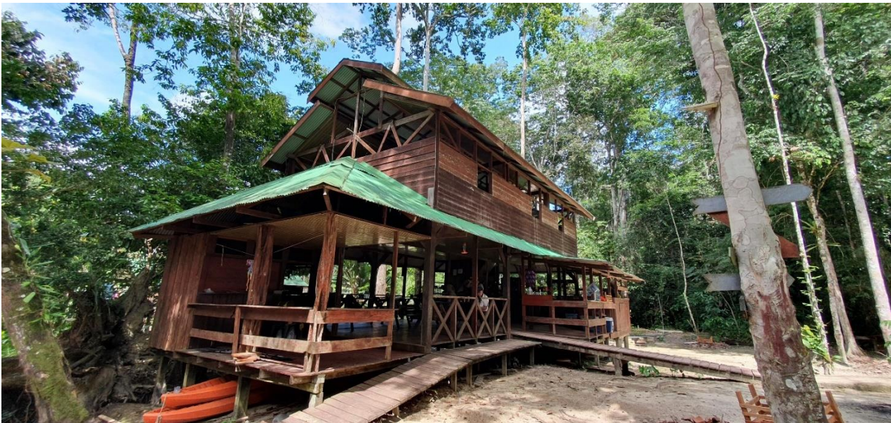
Zintete Lodge, on the ground floor the restaurant and on the first floor the communal dormitory (HG)
