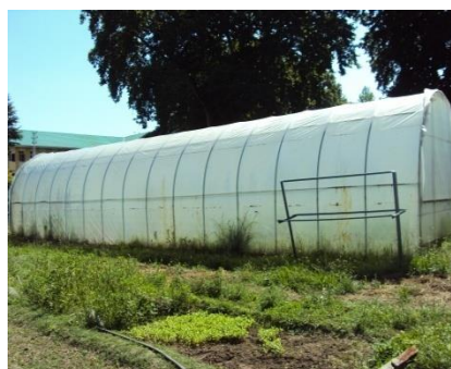
Fig. 9. Green house in University of Kashmir
