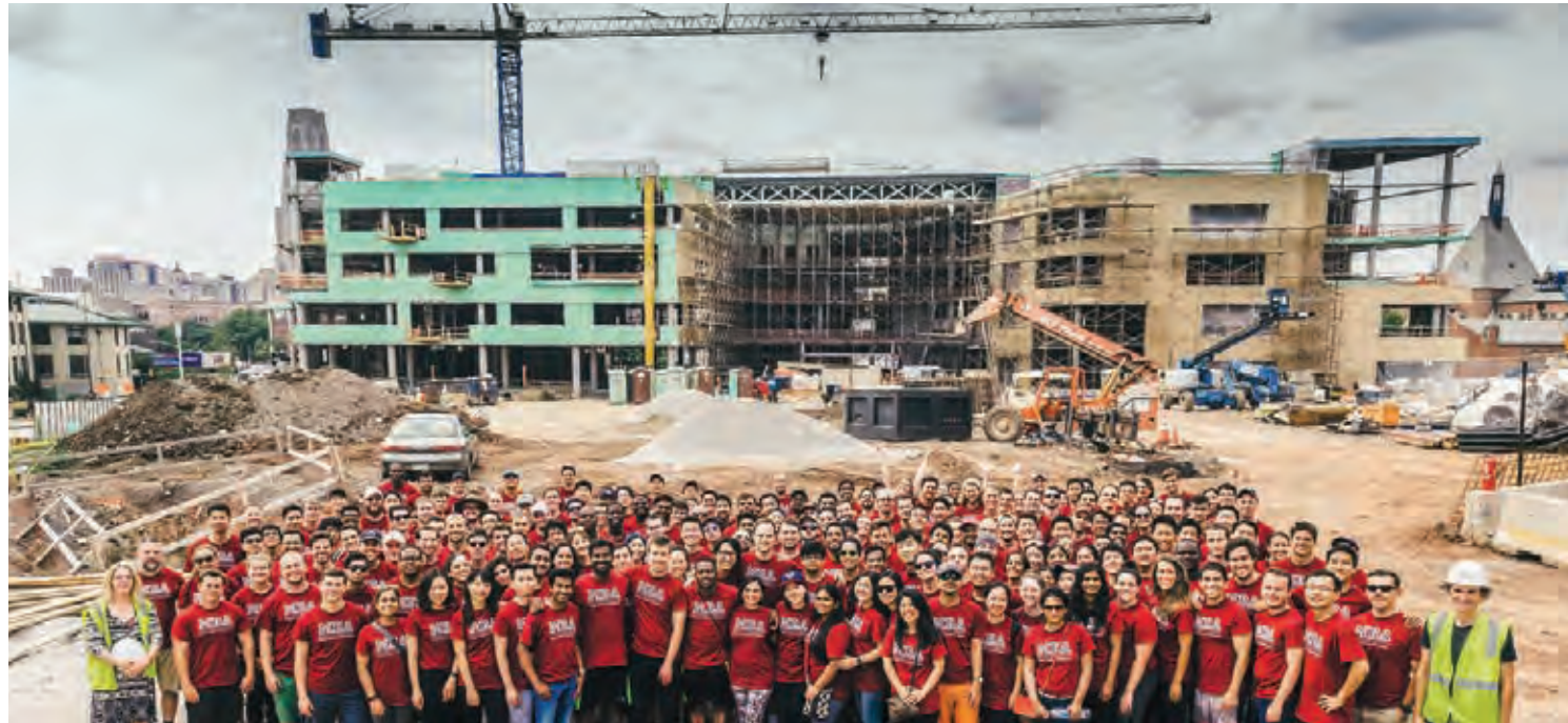
The Class of 2019 visits the construction site of the Tepper Quad, where they will spend their second year as MBA students.
