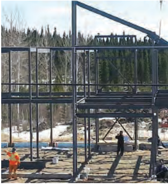
Building the Women Shelter in Waswanipi
