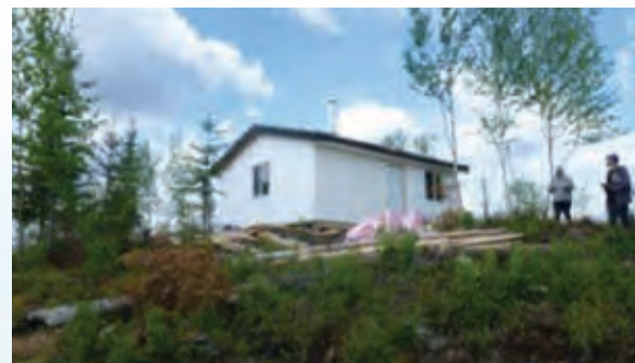
Cabin Construction through the Cree Traditional Activities Enhancement Program
