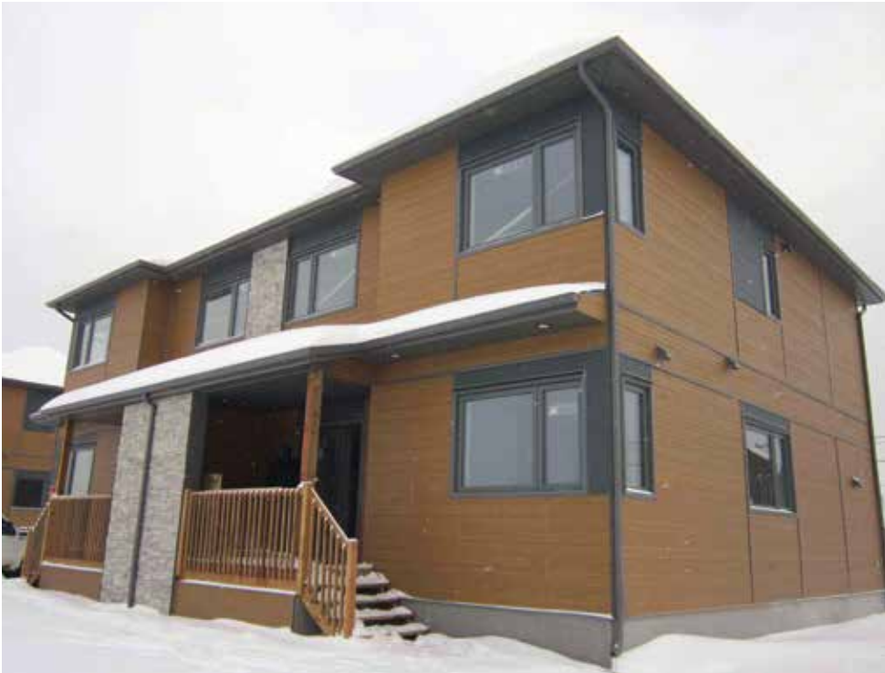
Top: Youth Custody Facility in Mistissini (in construction)
