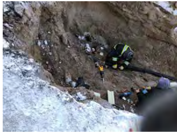
Chisasibi Operation Staff Performing Service Line Repair
