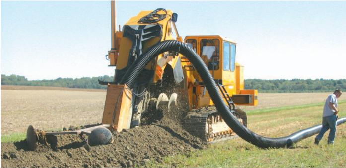
Figure 4. Installation of a modern drain tile made of lightweight, perforated plastic, in an agricultural field.
