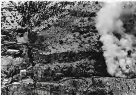
Fireballs. In the days that followed closure of the Wilberg mine, pockets of combustible gasses ignited sending spectacular fireballs chuffing from the entrance portal.
