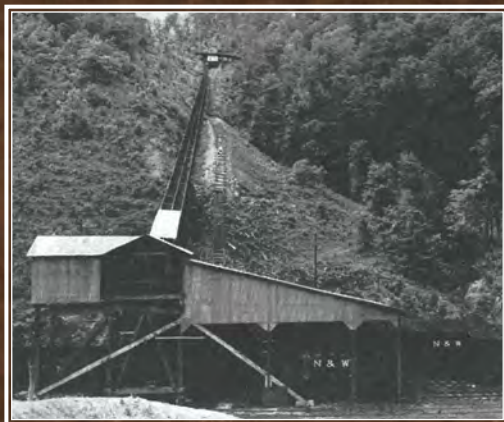
Home Creek Smokeless Coal Co. plant and retarding rope-and-button conveyor. This operation shipped the first coal from the Grundy field. * Coal Age , August 1934
