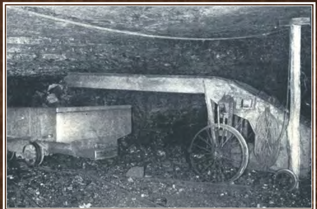
Brown-Fayer pit-car loader starting pocket in pillar, Cap Mine 32. * Coal Age , October 1930
