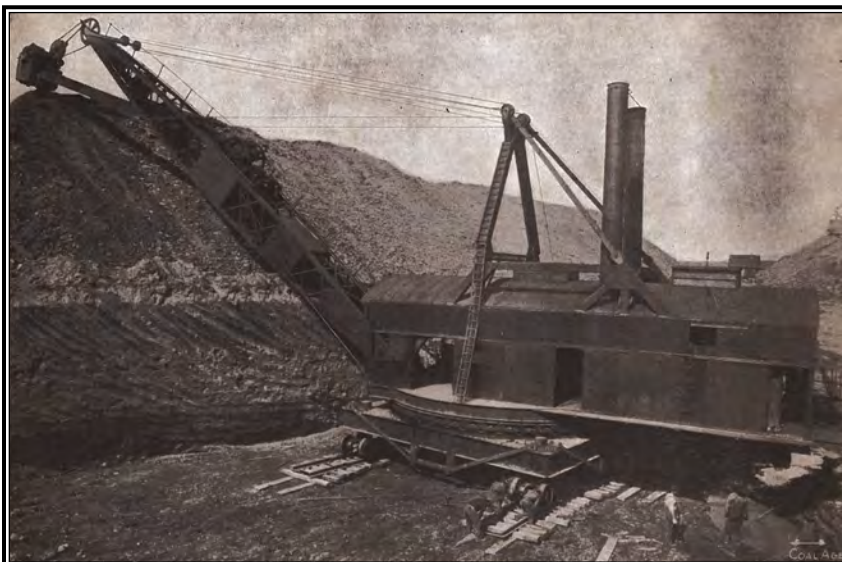
Photograph of the world's largest steam shovel on a stripping operation in Kansas. * Coal Age , January 4, 1913
