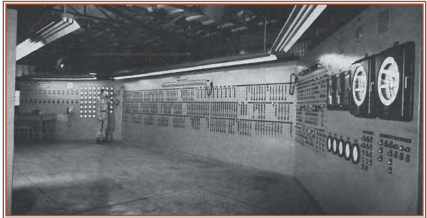
90% of machinery in the plant is controlled by a single operator. This 80-ft panel contains all pushbuttons, selector switches, indicating lights, ammeters, audible signal devices and other instruments for the washing portion of plant. * Coal Age , July 1959
