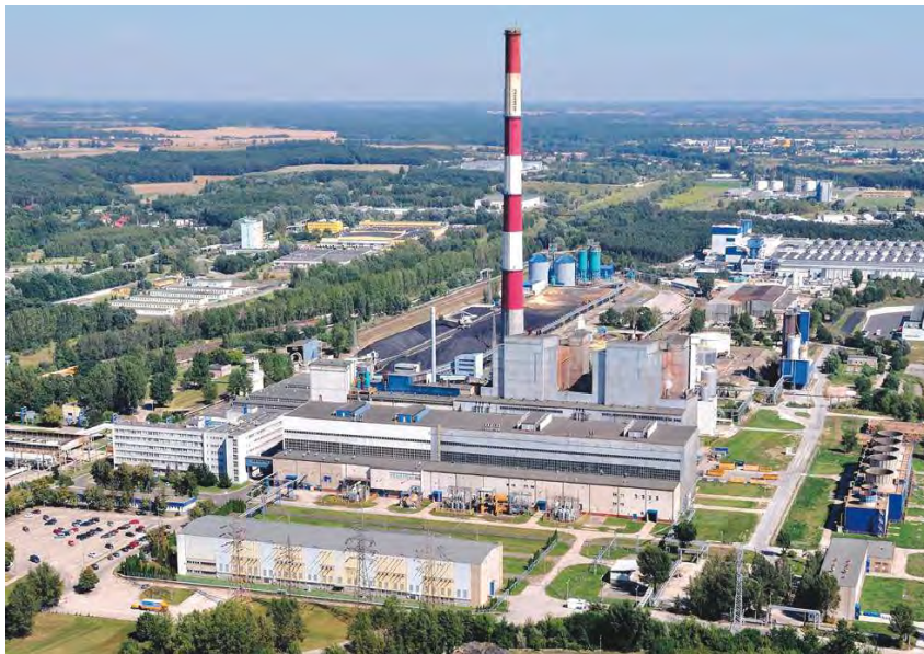
GE will upgrade one of three turbine-generator sets at Veolia Energia Pozna in Poland.
