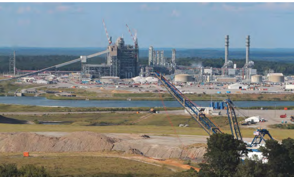
Duke Energy’s Edwardsport IGCC Project, above, with two gasifiers and engineered for eventual carbon capture for EOR, replaced a 160-MW pulverized coal-fired plant and came online in 2013. (Photo: Duke Energy)
