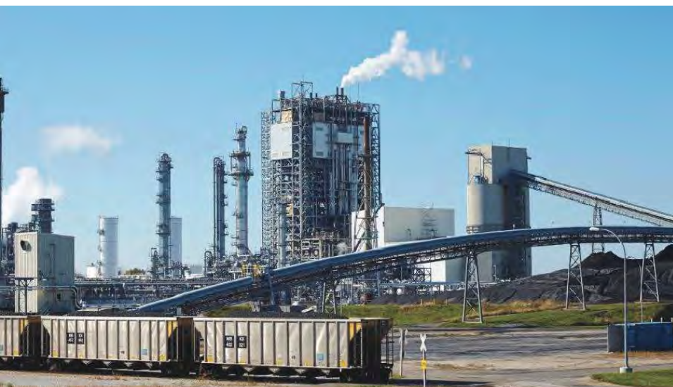
The biggest IGCC power plant in the world, Mississippi Power’s 582-MW Kemper County Energy Facility, above, features two gasifiers and captures CO 2 for enhanced oil recovery (EOR). It was reportedly operational in January. (Photo: Mississippi Power)
