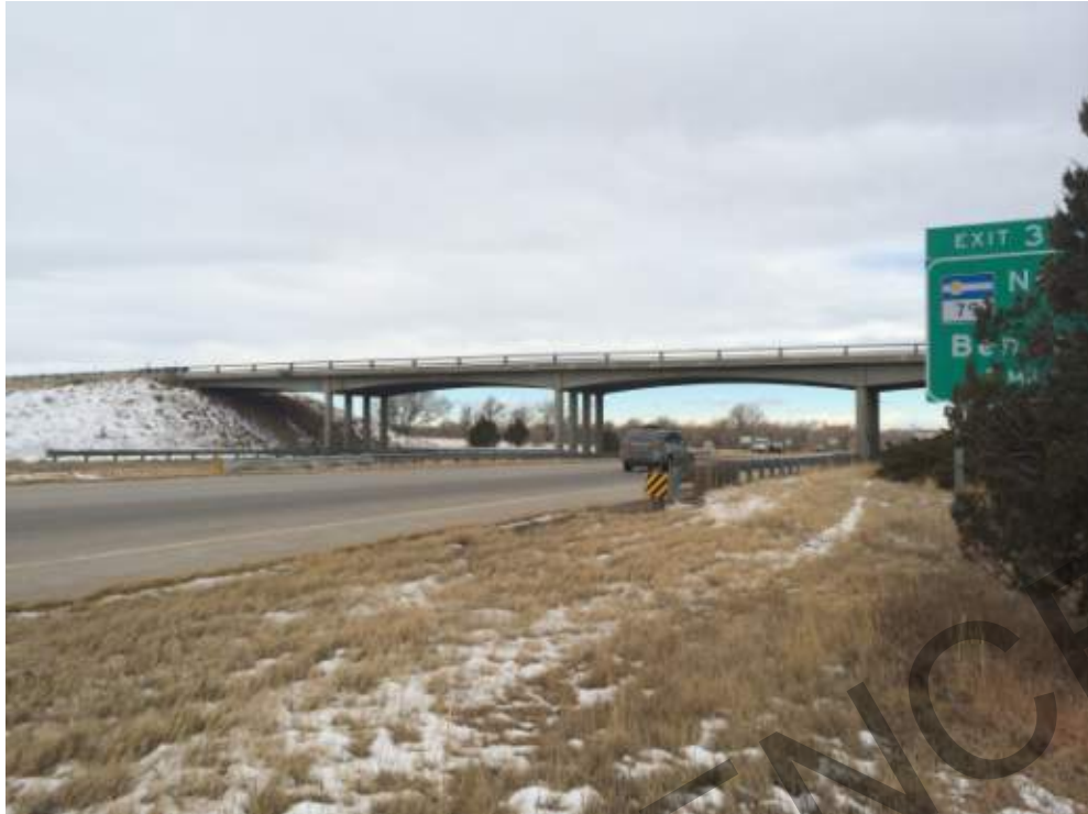
Photo 17 Looking East at bridge
