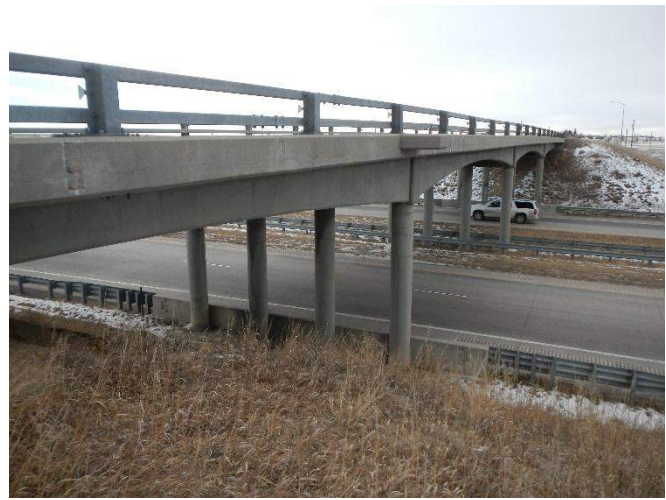
Bridge F-19-AF, view to the south-southeast.
