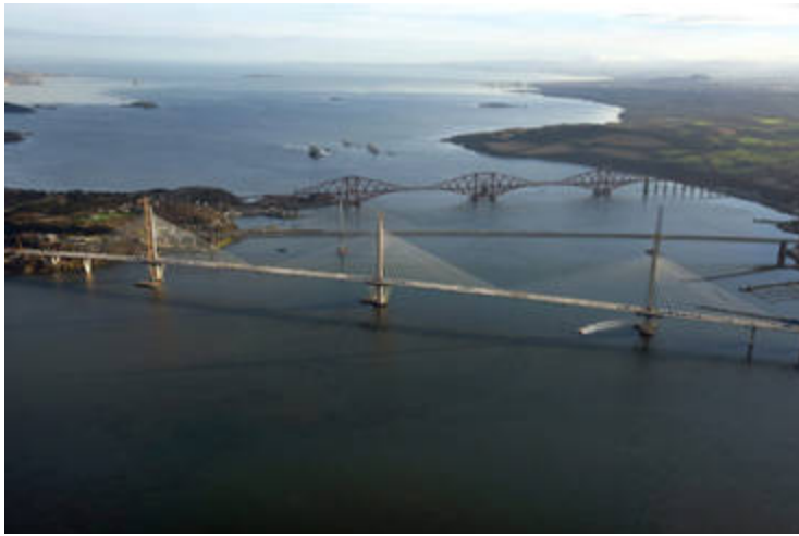
Fig. 1 - Forth Bridge, Forth Road Bridge, Queensferry Crossing Scozia (UK).
