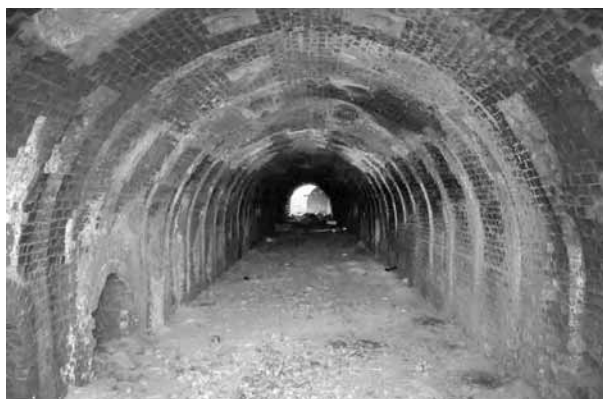
Interno camerette fornace Fusi
