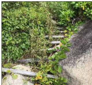
Stairs access from CTB (now removed)
