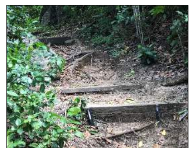
Eroded unsafe steps on the FB track
