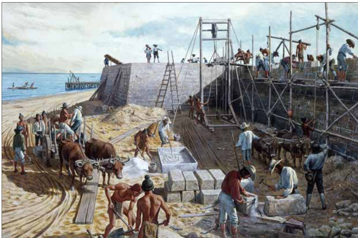
Spanish masons and an enslaved indigenous workforce built Fort Augustine with blocks of limestone.
