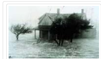
Storm surge swamps a house. (Photo: NOAA)
