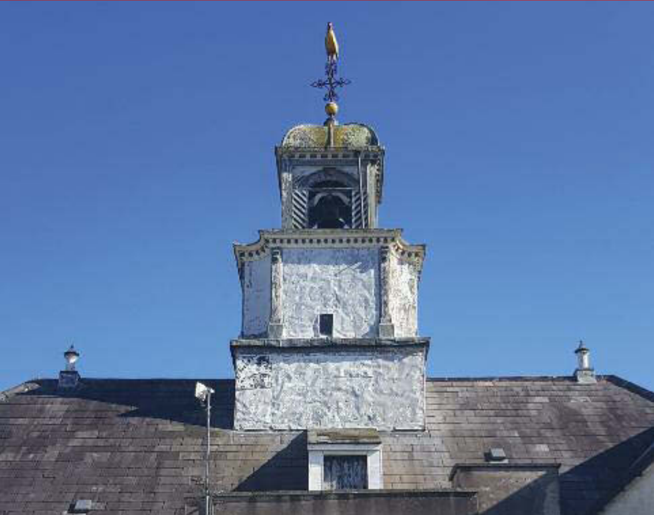
The roof of Midleton Library, Main Street, Midleton (2011). Image by Fourem.
