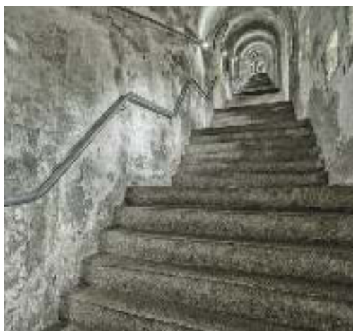
The underground vaulted staircase provided protective access between the upper and lower levels in the fortification.
