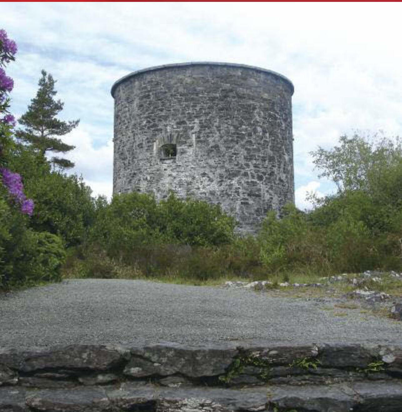
The Martello Tower on Garinish Island. Image from www.garinishland.com
