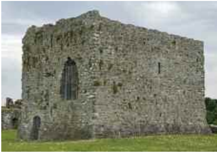
Central two storey Norman tower. Image courtesy of Pauline O'Dwyer.
