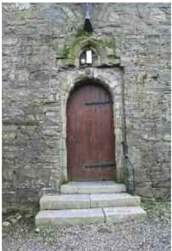
Door into tower.
