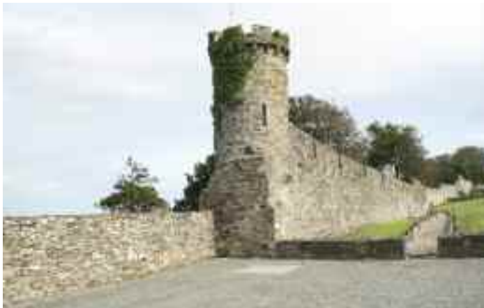
Section of the medieval Town walls, Youghal.
