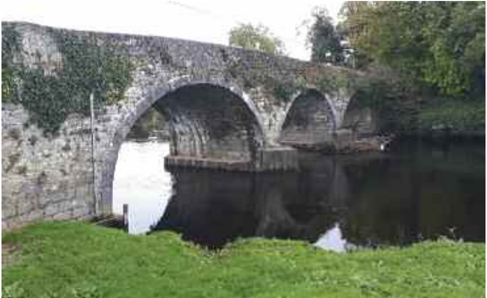
Killavullen bridge (CO034-00503).
