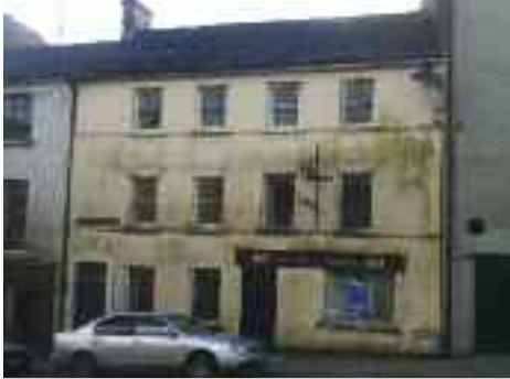
A 17th century house at 83 North Main Street, Bandon, concealed behind a 19th century façade
