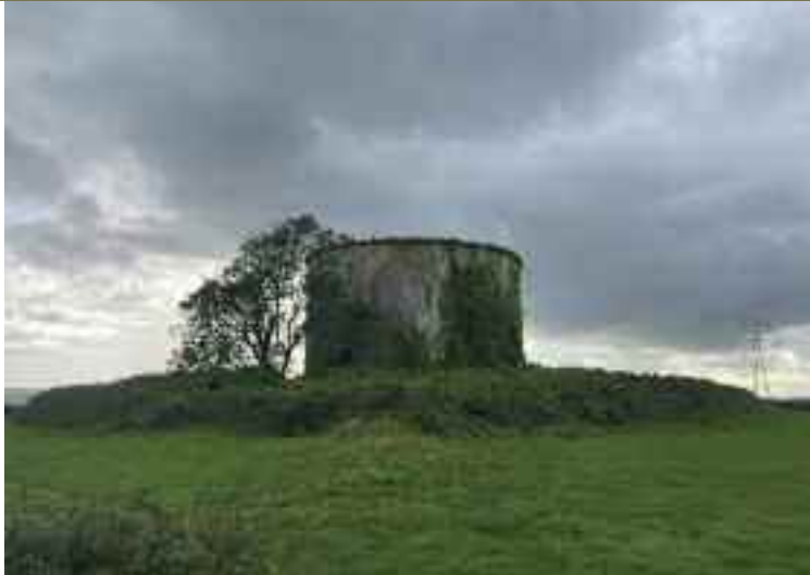
Ringaskiddy Martello tower. Image courtesy of Cllr Marcia Dalton.
