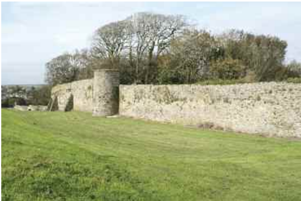
South west run of the town walls.
