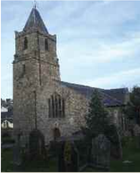
View of church from south west.
