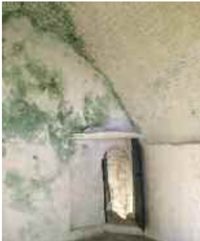
Wicker centred vault over third floor and pointed door to spiral stairs.
