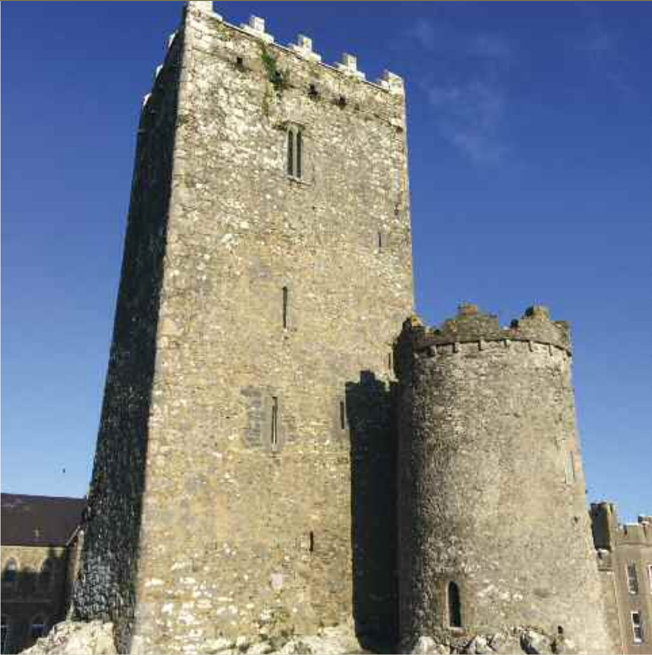
South elevation of the tower house.
