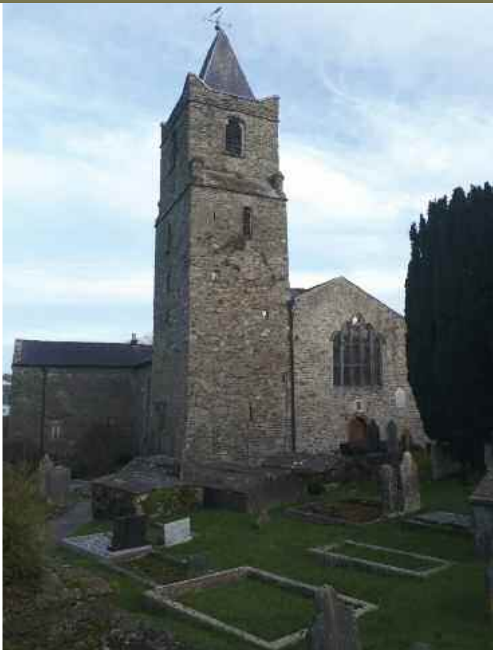
View of church from south east.
