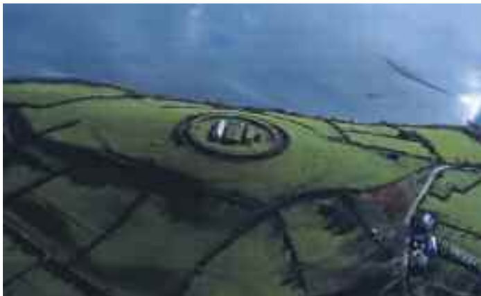
Central Redoubt (CO118-078), Whiddy Island, Bantry Bay.
