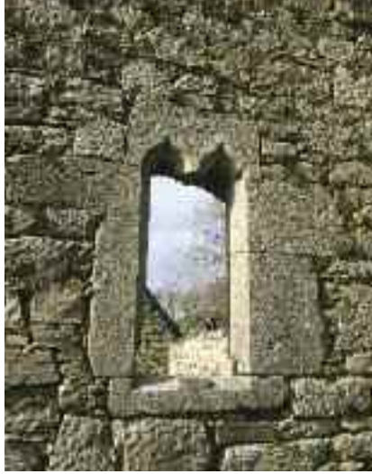
Ogee headed windows at Garryvoe Church (CO077-037002).
