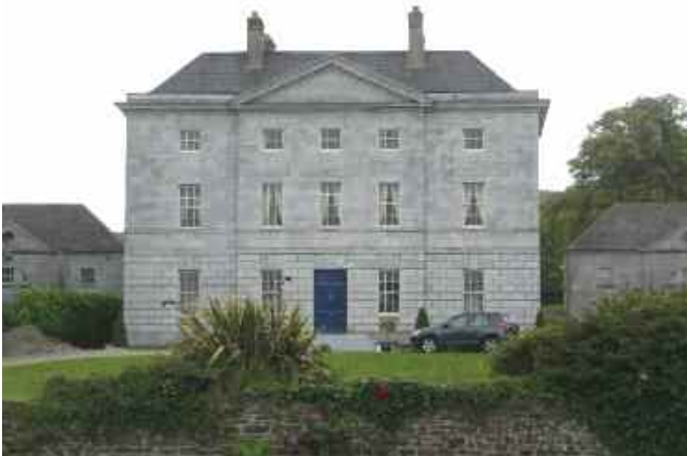
Crosshaven house (CO099-021)
