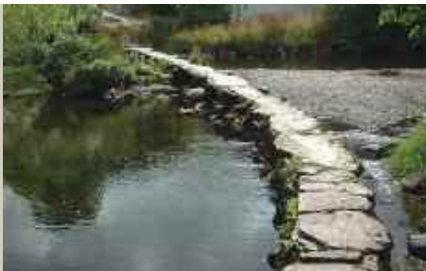
Ballingeary Clapper Bridge (CO081-008). Image courtesy of James Buckley.
