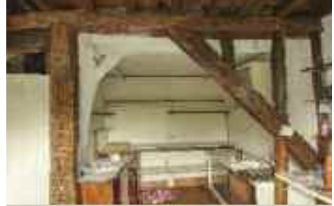
17th century timber frame inside 83 North Main Street, Bandon. The timbers were dated to 1659-1660 by dendrochronology in 2016, funded by the Cork Historical & Archaeological Society.
