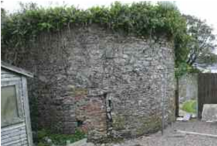
Banshee tower on the south west run of the town walls.
