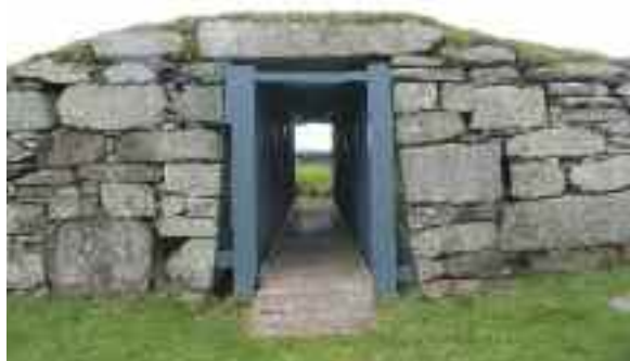
Stone-built entrance passage with supportive props.
