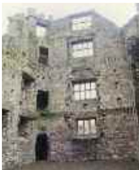
Interior showing floor levels and gun loops under large widows.
