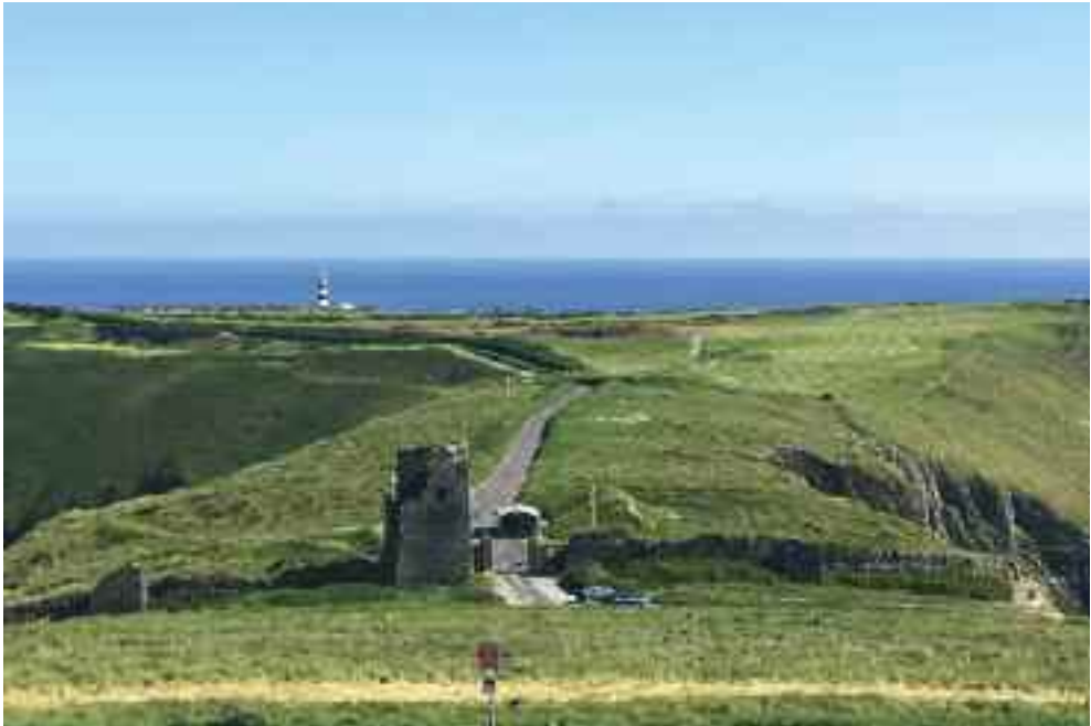
Old Head of Kinsale showing the external ditch (fosse) defences with the later medieval bawn wall and Tower house on top of ramparts. Image courtesy of Connie Kelleher.
