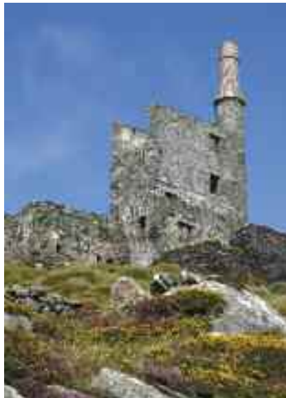
Engine Pump House at Allihies Copper Mines.
