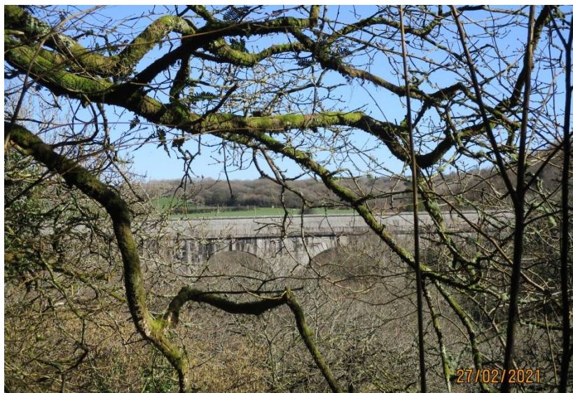
The Treffry Viaduct and aqueduct, built between 1839 and 1842.
