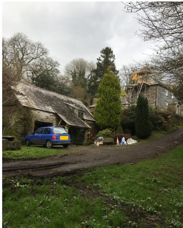
Battens Mill and mill house
