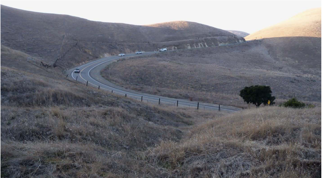
Viewpoint 6: View of the top of the grade on Tesla Road from the expansion area.
