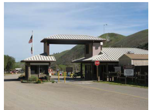
Carnegie SVRA entrance station
