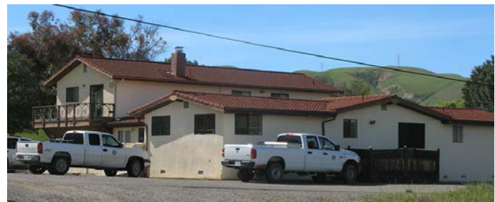
The Carnegie Sector office is located in a house left over from when the expansion area was used as a ranch
