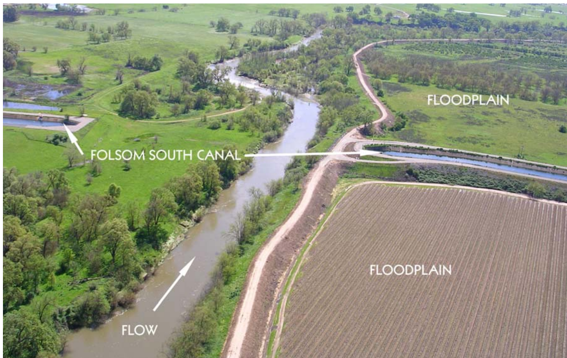
Figure 3-7. Aerial view of the Cosumnes River, floodplain, and Folsom South Canal looking west.
