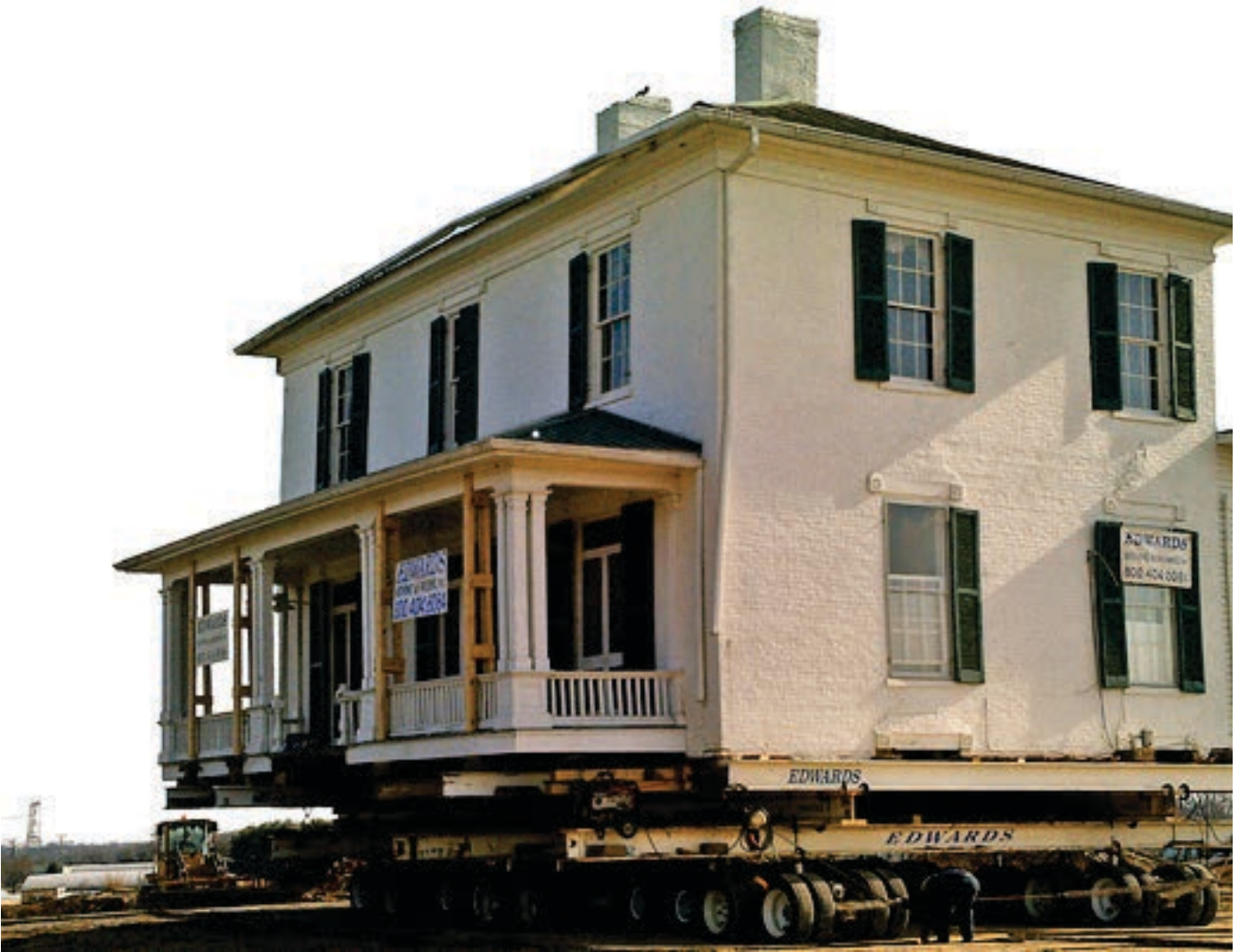
Example of building relocation
