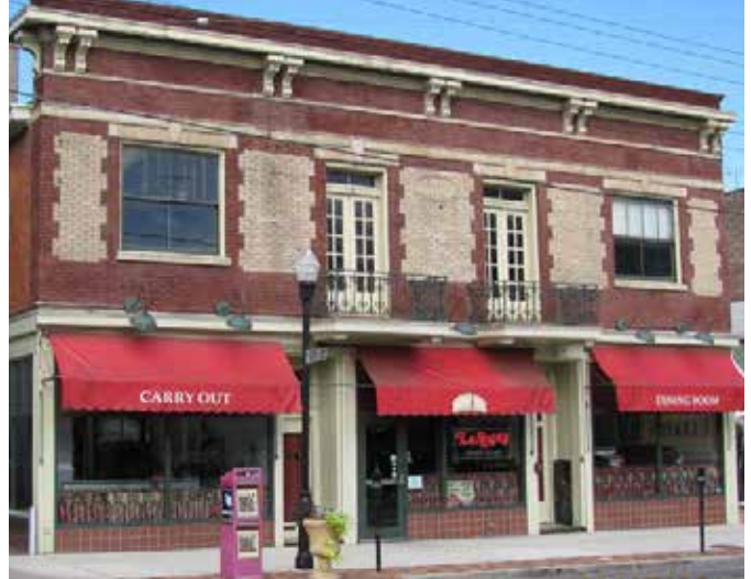
Example of an appropriate awning signage that received 7 points.
