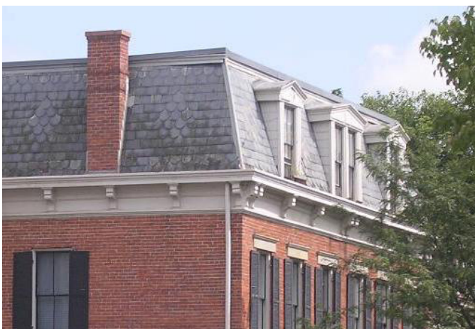
Mansard Roof with original slate shingle roof and dormers
