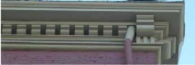
Example of an appropriately painted box gutter and downspout system
