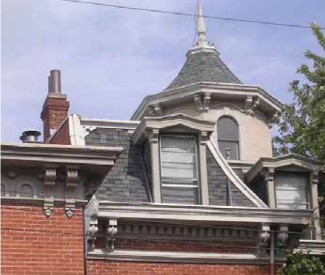
Examples of dormers, chimney, cornice, and eaves
