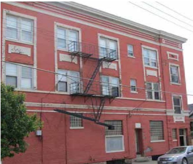
Example of fire escapes
