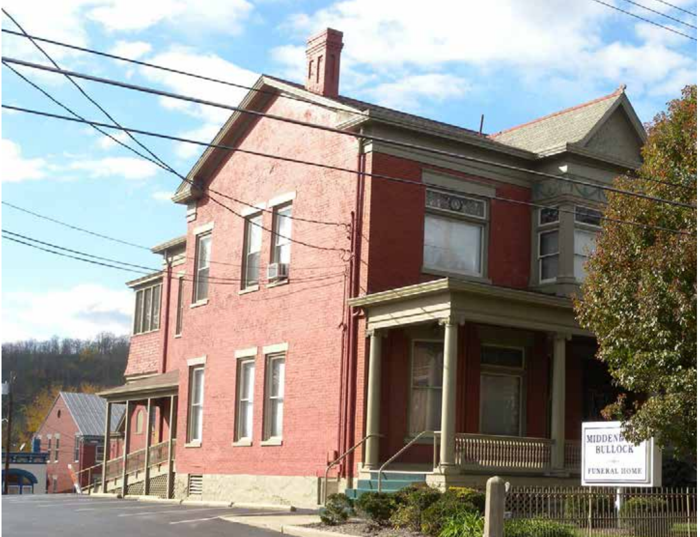
Example of accessibility ramp on the rear of a building
