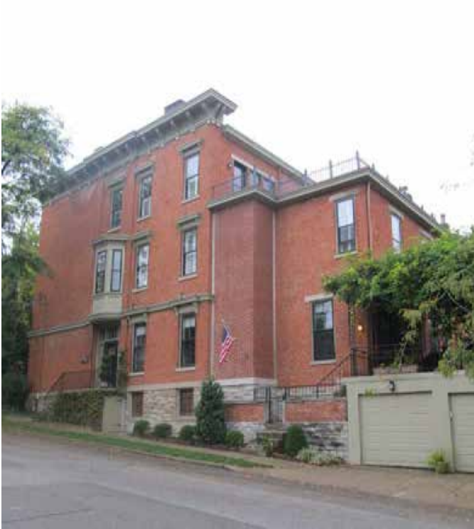
Example of an elevator addition on the side of a building
