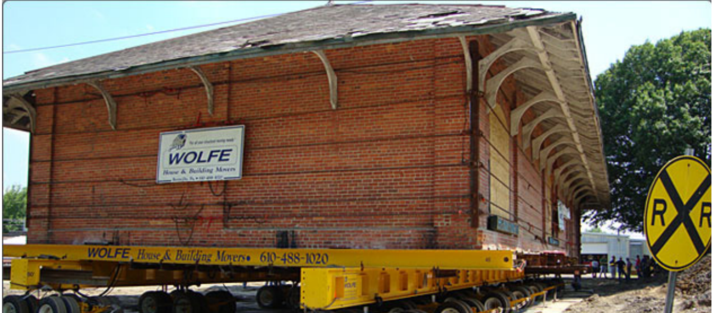
Example of building relocation
