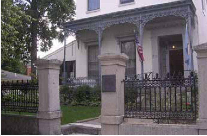
Example of decorative iron work fencing and a metal balcony
