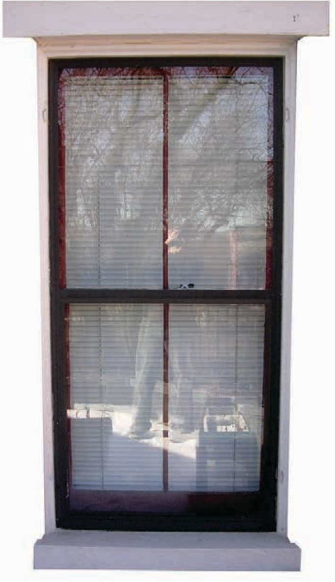
Example of appropriate storm window
