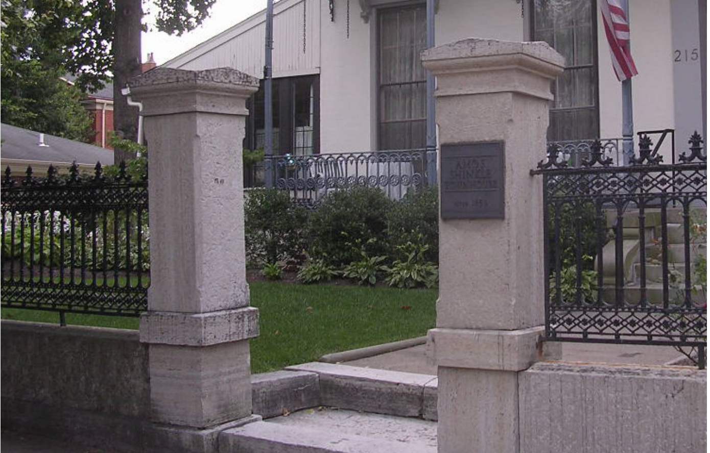
Examples of decorative iron fences in the front of buildings
