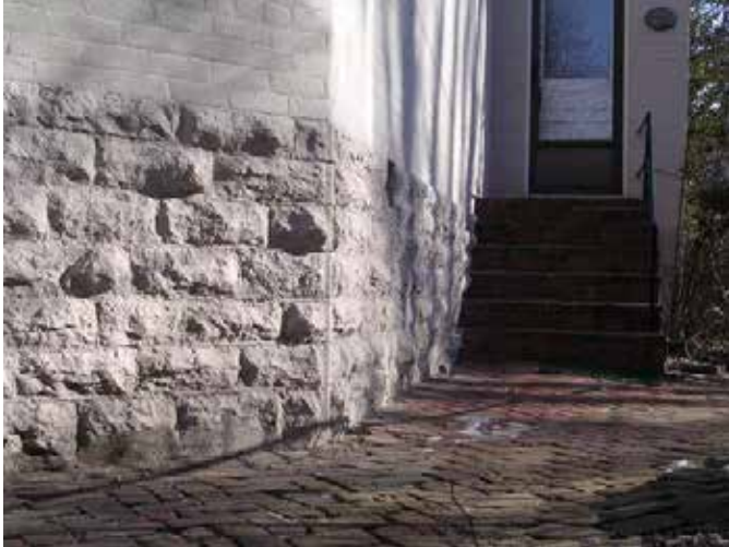
Example of a masonry foundation and brick walls in good repair
