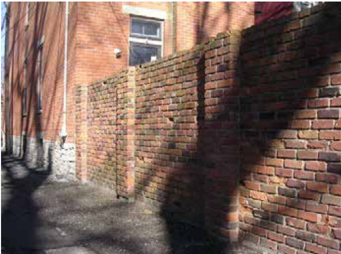
Example of brick privacy wall
