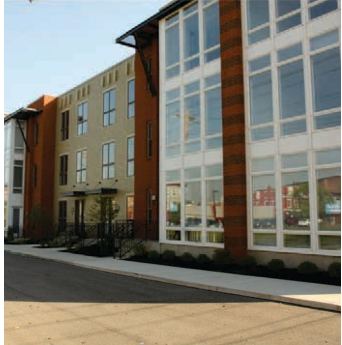
Example of infill on Banklick Street that used a similar materials fenestration rhythm and height of other buildings found within the neighborhood.
