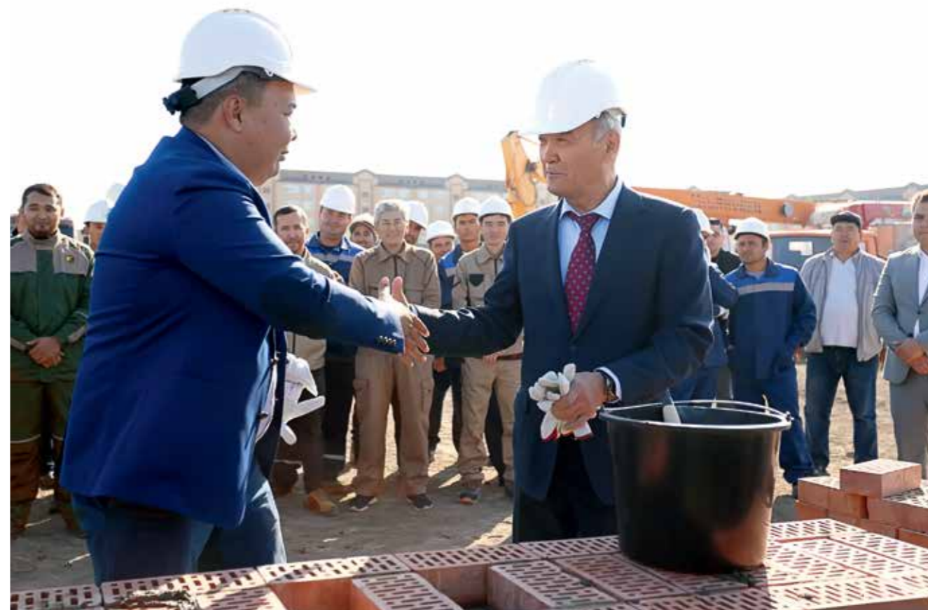
AT THE START OF THE CONSTRUCTION OF A SCHOOL IN THE TALGAIRAN MICRODISTRICT. 2022
