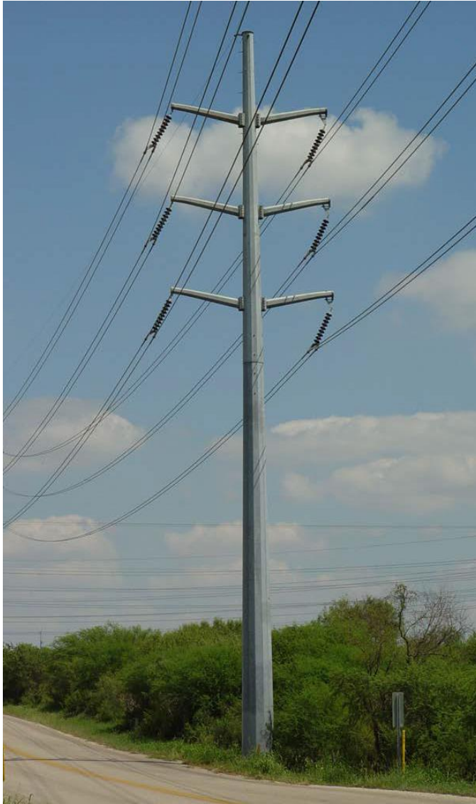
Figure 3. Typical steel monopole transmission line.
